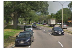
Vehicles are shown parked over the edge line of the shoulder, and doors extend into the lane when opened.
