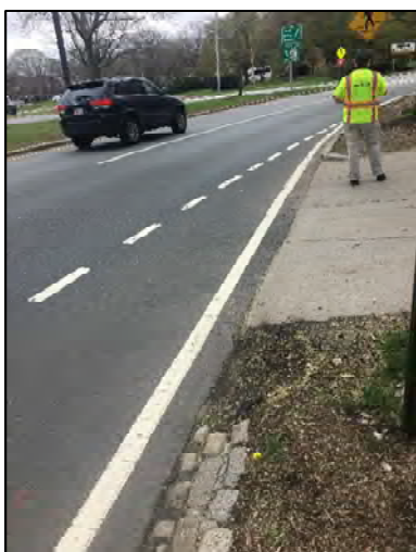
Bicycle lanes taper at the Carriage Road southbound approach to the rotary.
