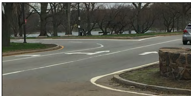
The pavement markings indicating lane use is provided after the motorist's decision point.
