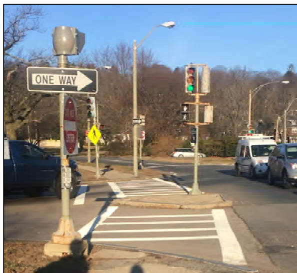
The signalized crossing across Arborway at Centre Street does not have ramps or pedestrian head with countdowns.
