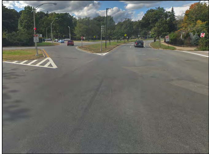
The signal facing the Centre Street eastbound approach is visible to the Arborway northbound traffic.
