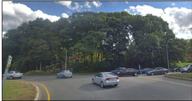
Lane usage is not clear in Murray Circle causing many motorists to drive in the middle of one wide travel lane.
