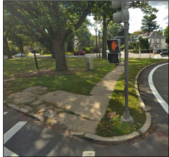
The pedestrian signals at the Arborway northbound entrance to the rotary are outdated, and the wheelchair ramps are in poor condition.
