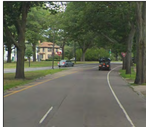
The Carriage Road merges from two lanes to one lane with no warning for motorists.
