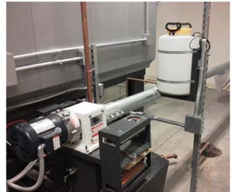
An auger injects pellets into the boiler
