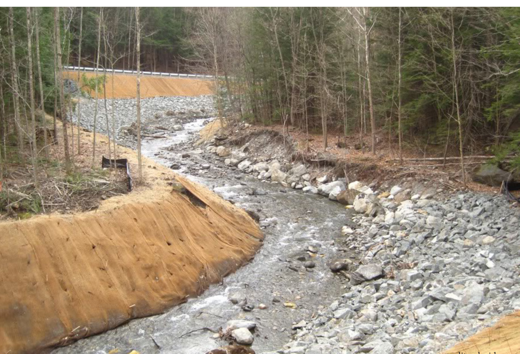
Shown here in 2012, Clesson Brook sustained significant erosion from Tropical Storm Irene. The riverbed was reconstructed in several places to increase stability.
