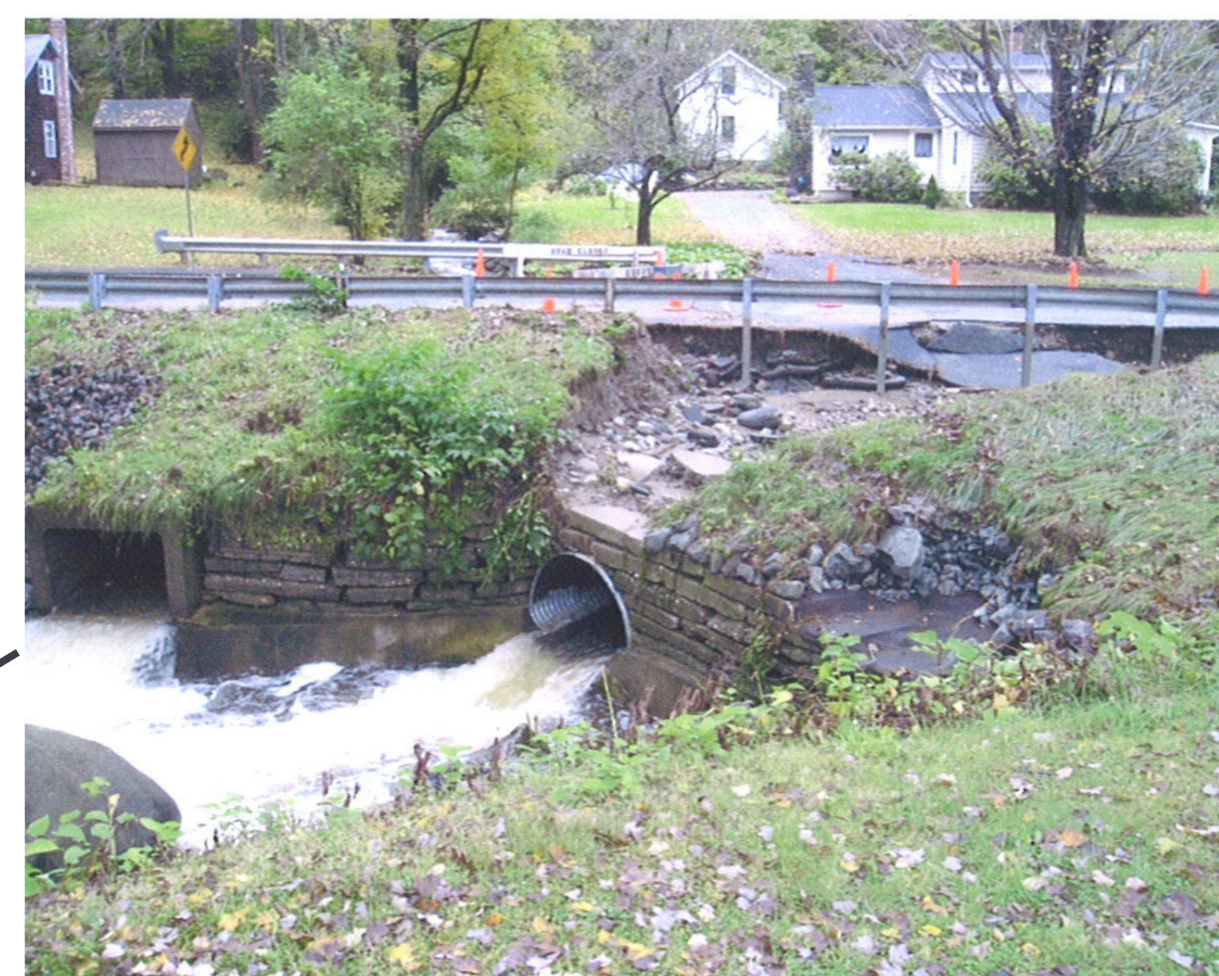
Shown here in 2005, the South Street culvert, among others, is in need of repair. Extreme weather events can erode and damage culverts leading to flooding and unstable roadways.
