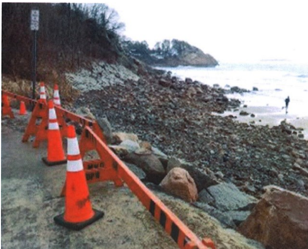
Singing Beach, Manchester-by-the-Sea. The roadway, structures and revetment have been damaged a number of times and repaired by the Town at significant cost. The damages shown above were from the winter of 2013.
