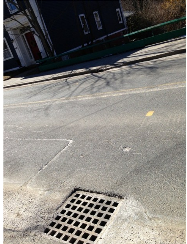
Storm Drainage system on School Street with direct discharge to Sawmill Brook
