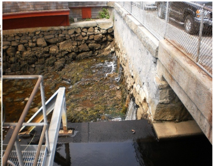
Seepage at the seawall.
