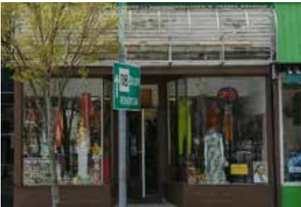
The awning framework remains, needing a new material cover or removal.
