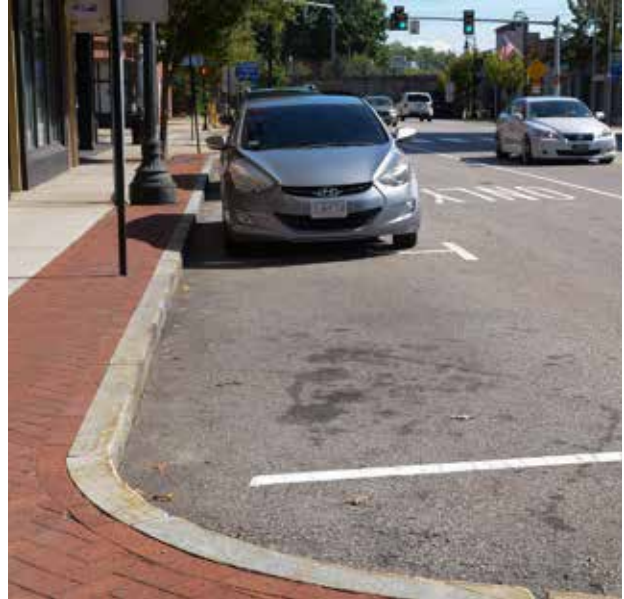
Parking pavement markings delineate the length and width of a parking space on South Main Street.
