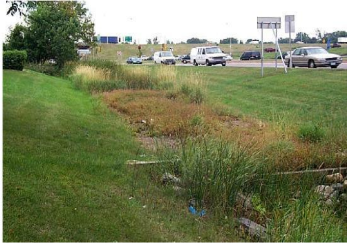
Figure B.13 – Photograph of water quality swale
