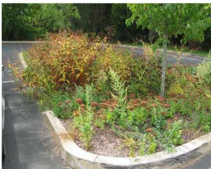
Figure B.1 Picture and schematic of bioretention
