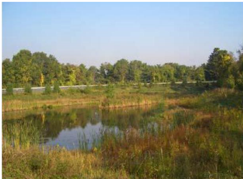
Figure B.3—Photograph of constructed stormwater wetland.
