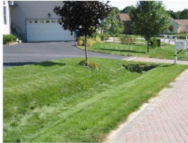
Figure B.12—Photograph of vegetated drainage ways.
