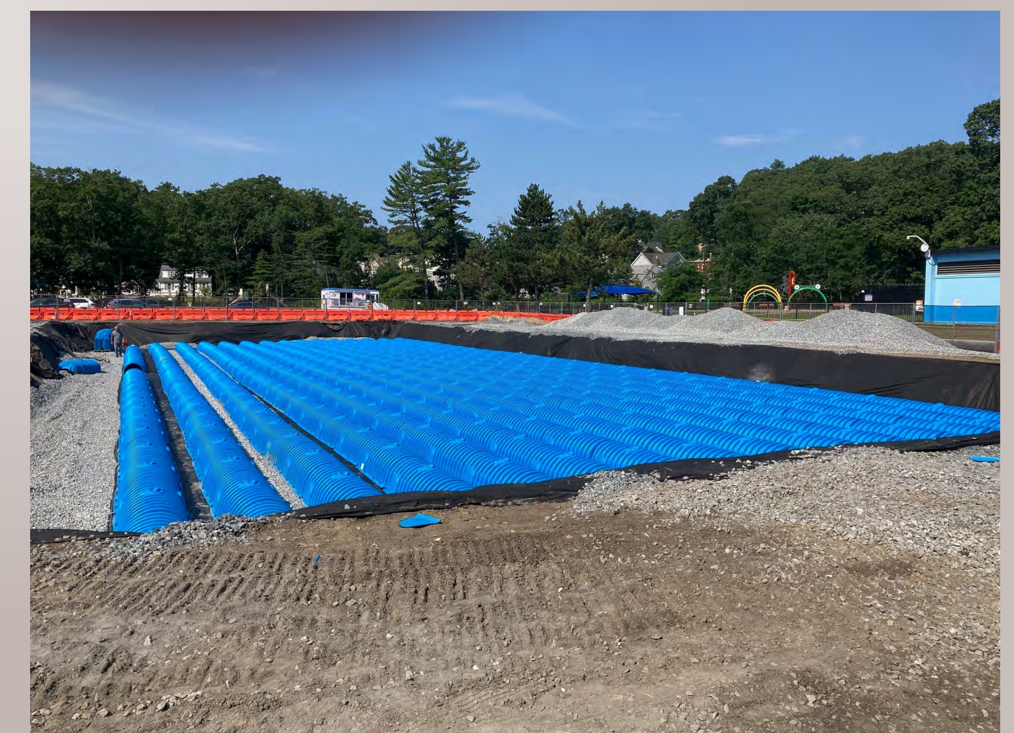
Construction of Underground Infiltrator Units
