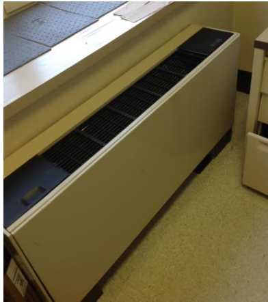
Photo 2 – Representative Unit Ventilator
