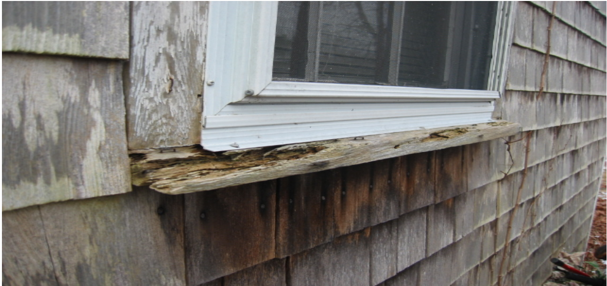
705-1 Development, 227 Sea Street Shingles Are Weathered and Decaying
