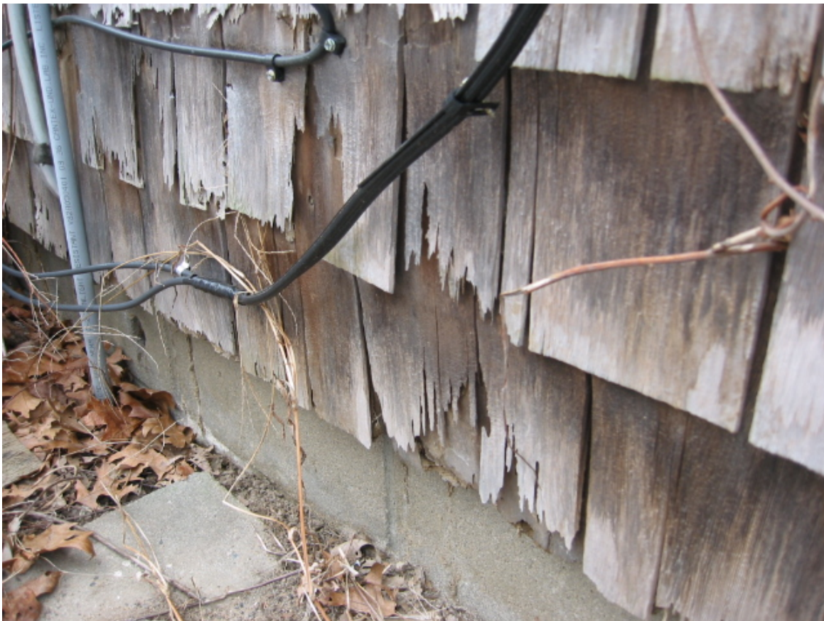
705-1 Development, 227 Sea Street Shingles Are Weathered and Decaying
