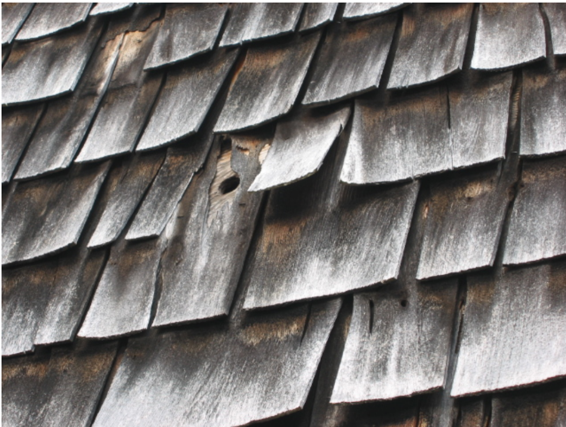
705-1 Development, 131 LaFrance Road Holes in Shingles, Breaking and Curling Upward
