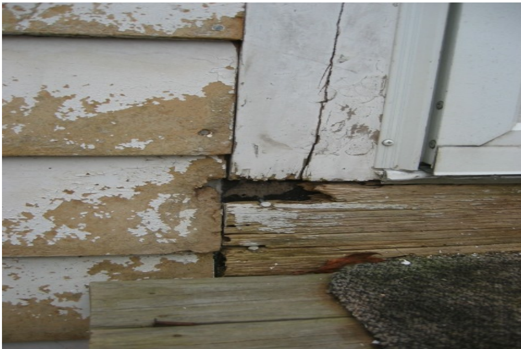
705-1 Development, 164 Arrowhead Drive Water Damage under Door, Rotted Threshold
