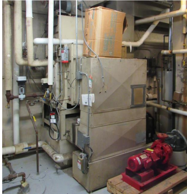
Photo 2 – Air handler AHU-1
