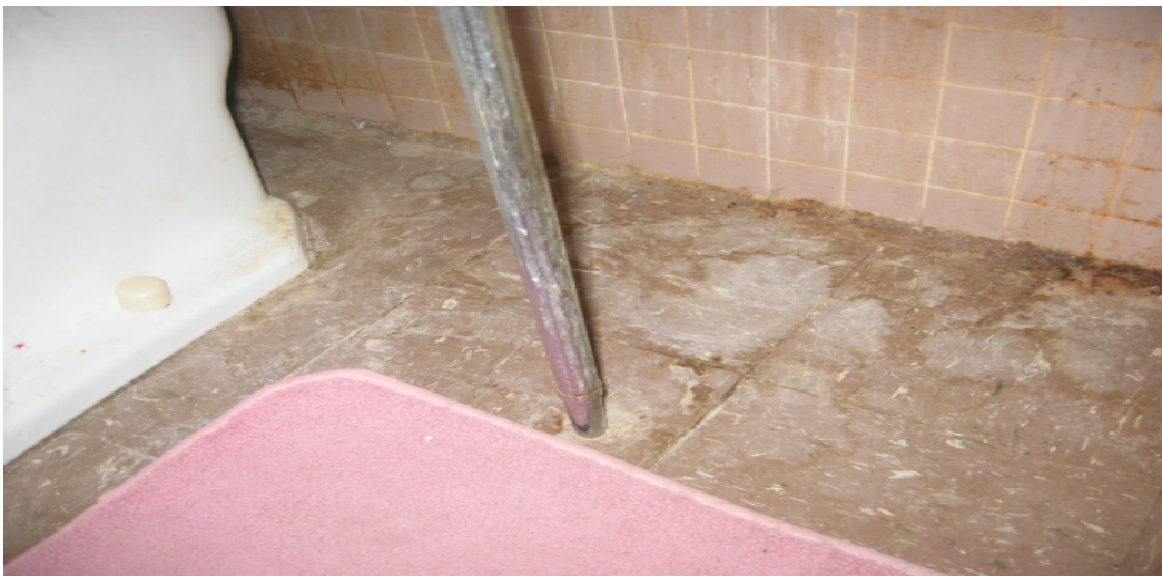
667-1 Development Ashby Circle, Building B, Apartment 8 Water and Mildew Stain on Bathroom Floor
