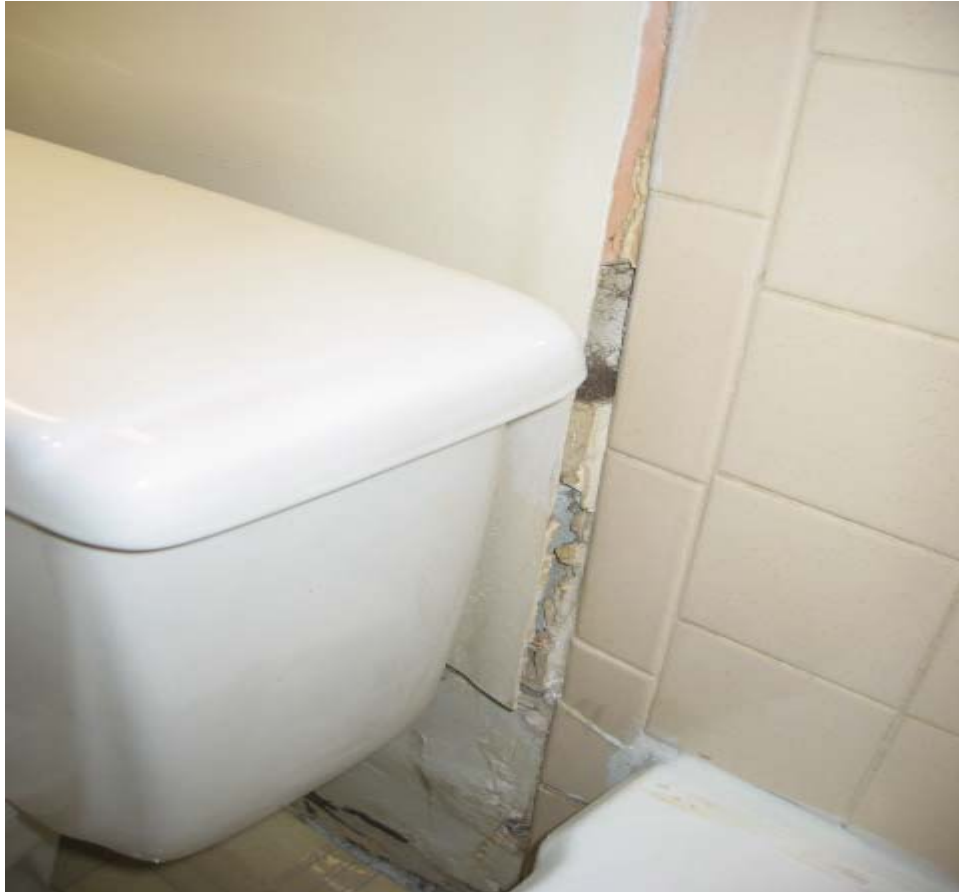
667-1 Development Ashby Circle, Building B, Apartment 8 Water and Mildew Stain on Bathroom Floor
