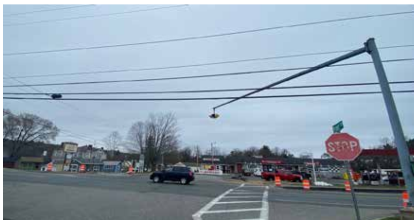
Intersection of Rte 202 and Stadler Street
