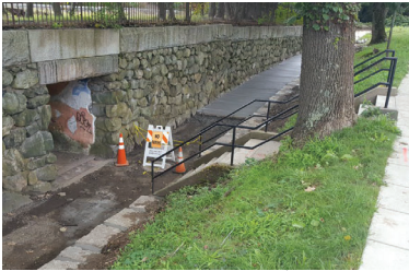
New walkway and drainage improvements near the Belmont Center Commuter Rail on Concord Ave. Photo credit: town of Belmont, 2018, via Twitter.
