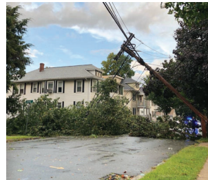
Downed tree and power lines. Photo by Belmont Light, 2019, via Twitter.
