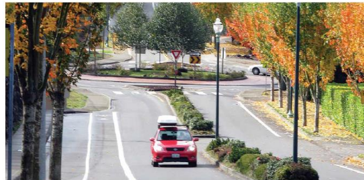
Vehicle speeds on Grandview Drive in University Place, Wash., often reached or exceeded 50 mph. After the installation of modern roundabouts, vehicle crashes dropped from one every nine months to zero in 14 years.
