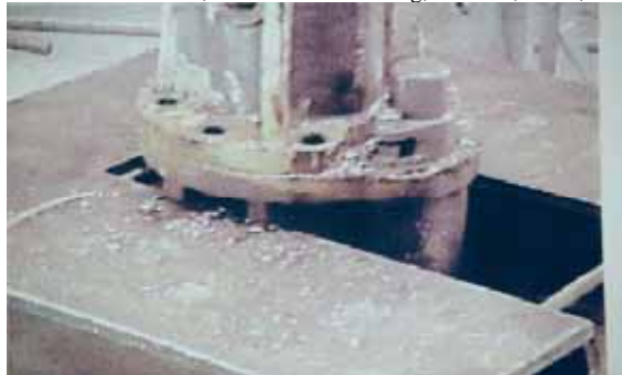
FIGURE 1: MERCURY SPILL AT PUBLIC WATER SYSTEM FROM MERCURY SEAL
