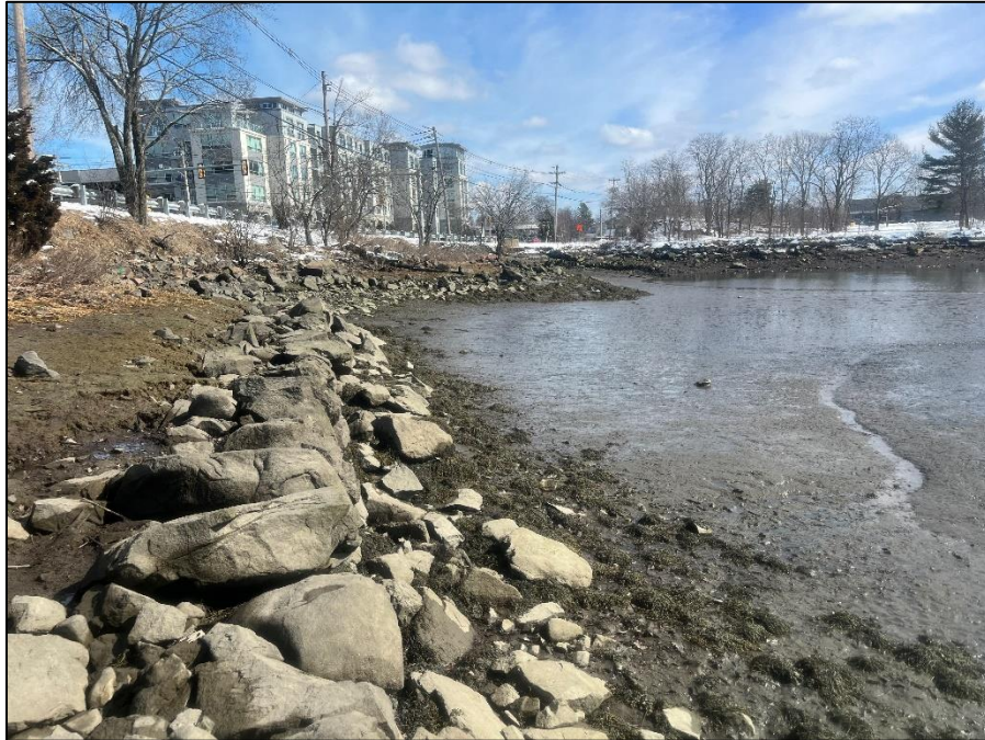
Figure 14. Fringing, rock-sill-supported salt marsh on the north shore of the upstream basin.
