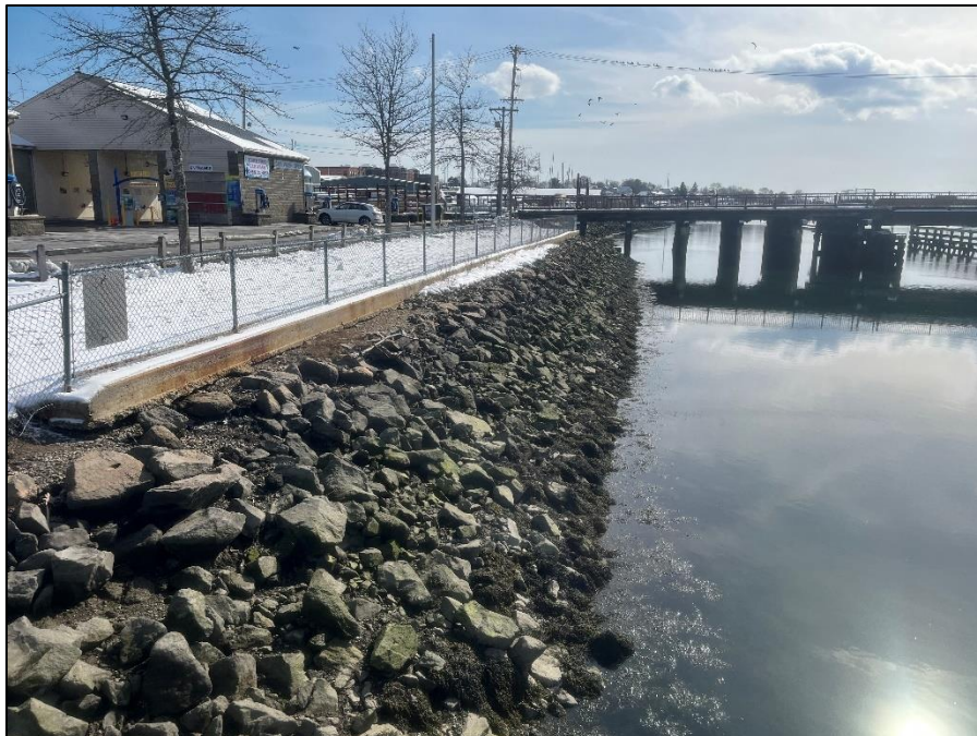
Figure 12. Rock revetment north of the Bridge Street bridge. Photo taken facing south.
