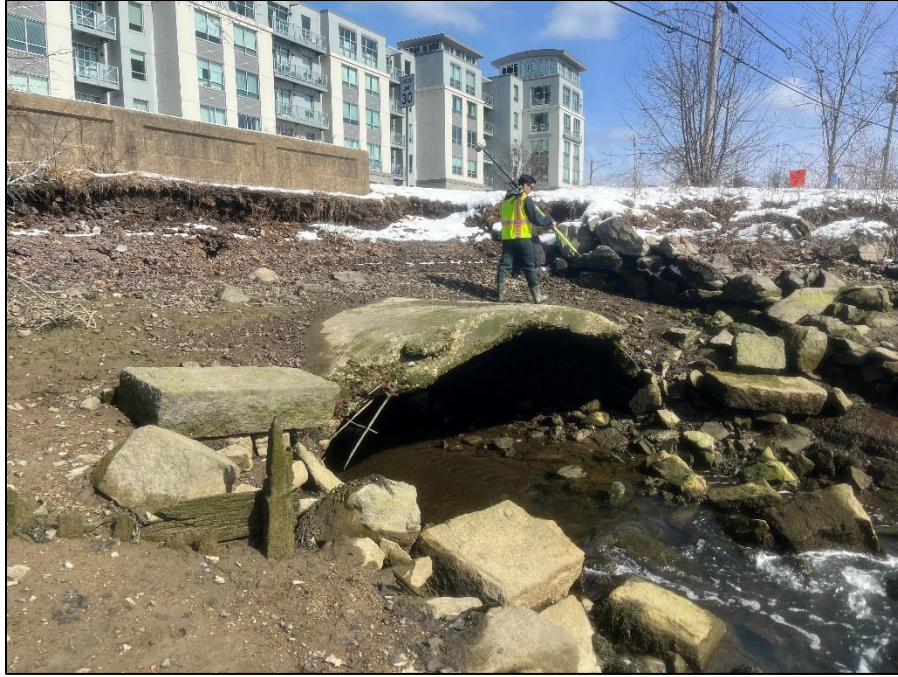
Figure 5. Coastal bank erosion extending landward to the roadway abutment along Elliott St.
