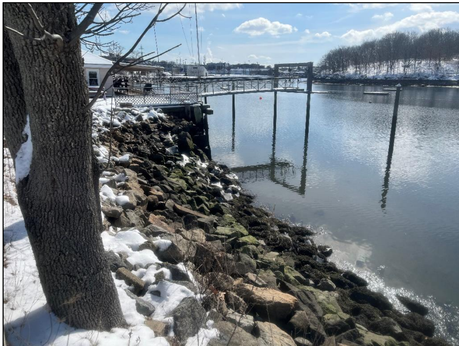
Figure 8. Sloping rock revetment seaward of boatyard. Photo taken facing south.
