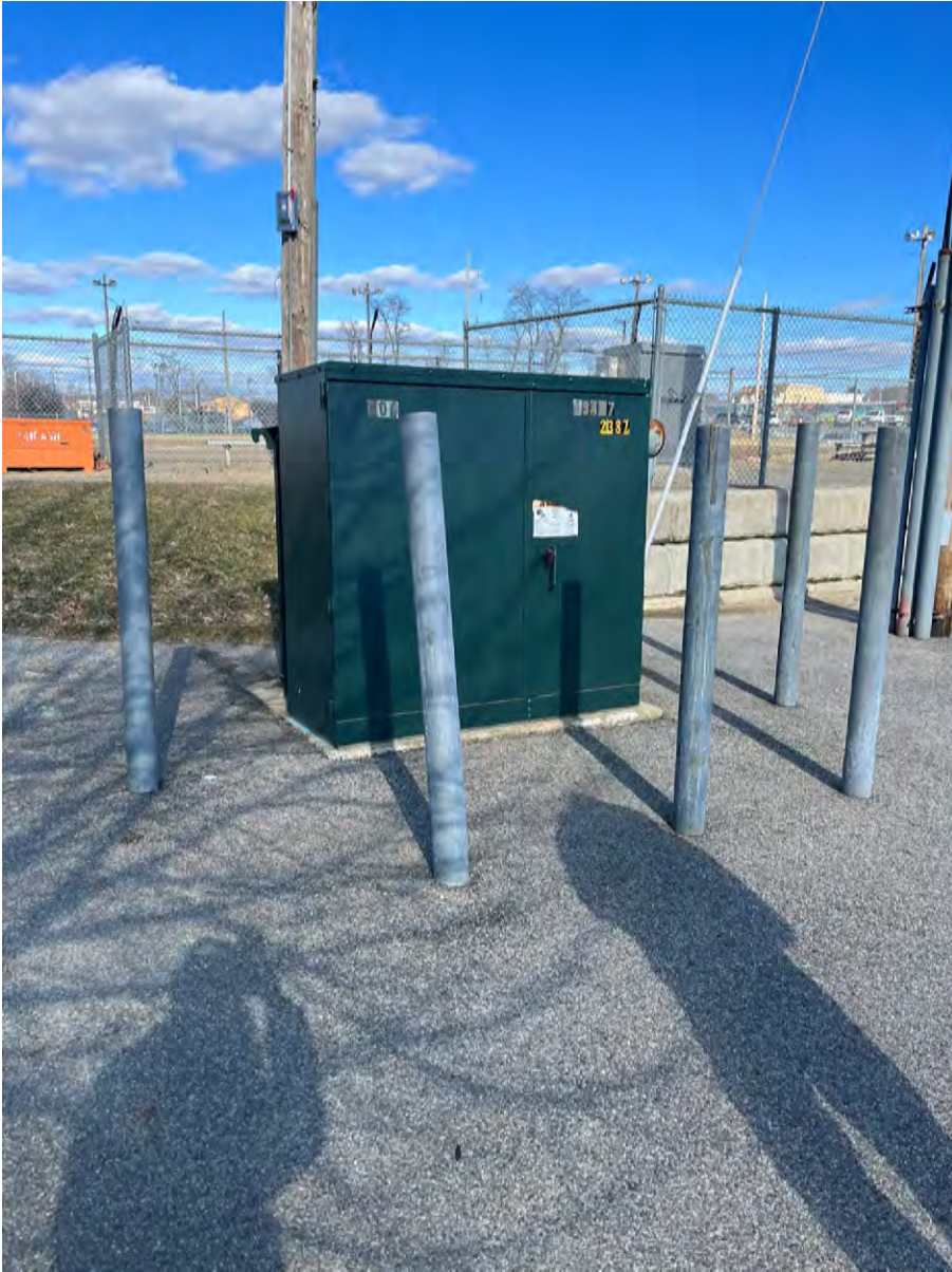
Photo 1: Ground Mounted Transformer
