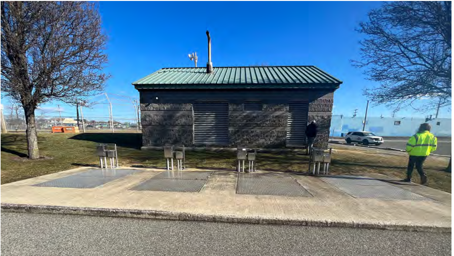
Photo 3: Pump Well Hatches (4)
