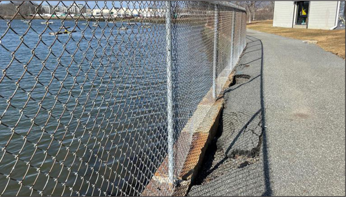
Photo 6: Stormwater damage adjacent to McPherson Youth Center
