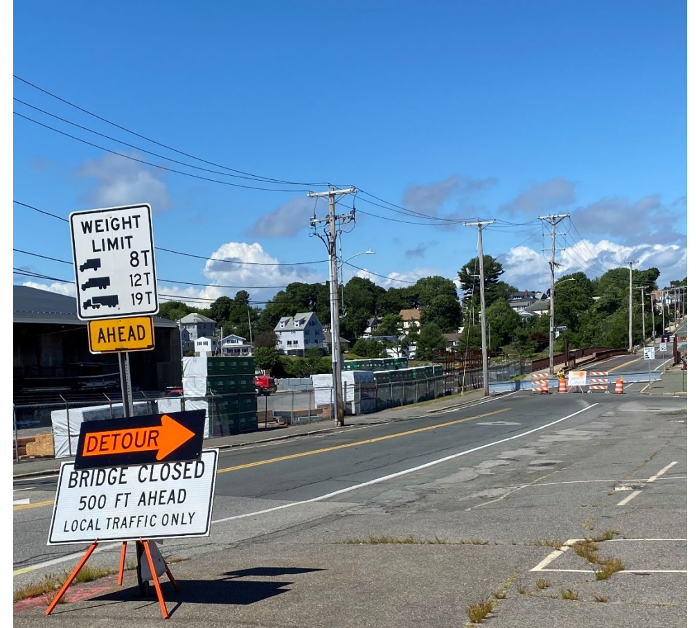
Existing Bridge Closed to Traffic
