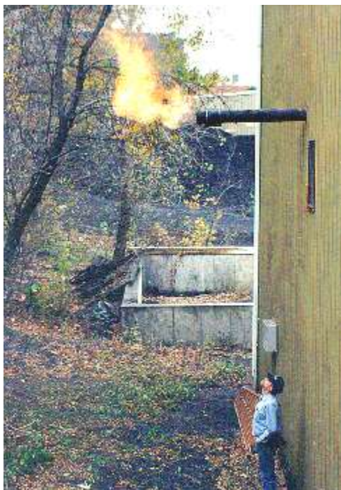
Figure 2-1. Gas Flare from an Experimental 5 TPD Biomass Gasifier.
