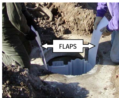
Step 2: Insert Liner
