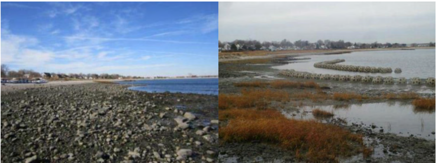
Figure 6. Stratford Point, CT Bioengineered Shoreline Restoration using reefballs and native saltwater marsh plantings. On the left is the original shoreline prior to the installation of the bioengineered shoreline stabilization measures. The photo on the right shows the same site following project completion. (Source: J. H. Mattei)
