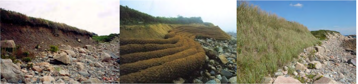
Figure 5. Massachusetts bioengineered coastal bank restoration. On the left the pre-intervention condition is seen. In the middle image, coir logs are installed along eroding shoreline. The photo on the right shows the same site ten years after project completion. The established native vegetation has stabilized the bank face. (Source: https://climateactiontool.org/content/restore-natural-coastal-buffers-bioengineering-coastal-banks )
