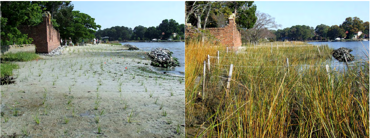
Figure 4. Sand fill with stone sills and marsh plantings at the Hermitage Museum, Norfolk VA. The image on the left shows the site just after completion of the marsh sill project and on the right, the same location after the vegetation had begun to establish itself. (Credit: W. Priest)
