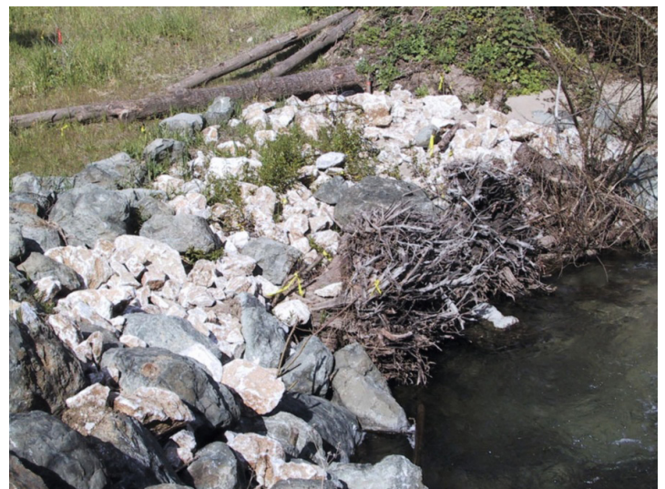
Figure 3. San Vicente, CA: Rootwads and Revetments (Source: Goldsmith et al. 2014)
