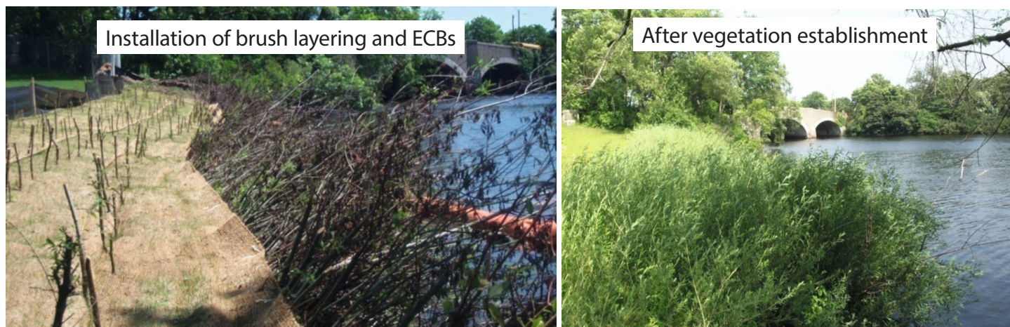
Figures 8 & 9. Charles River, MA Watertown Arsenal Bioengineered Streambank Restoration (Source: Goldsmith et al. 2014)
