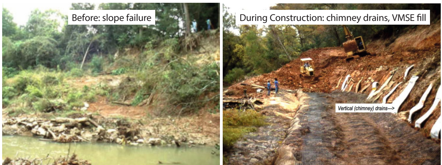
Figures 6 & 7. Buffalo Bayou, TX Bioengineered Streambank Restoration (Source: Goldsmith et al. 2014)
