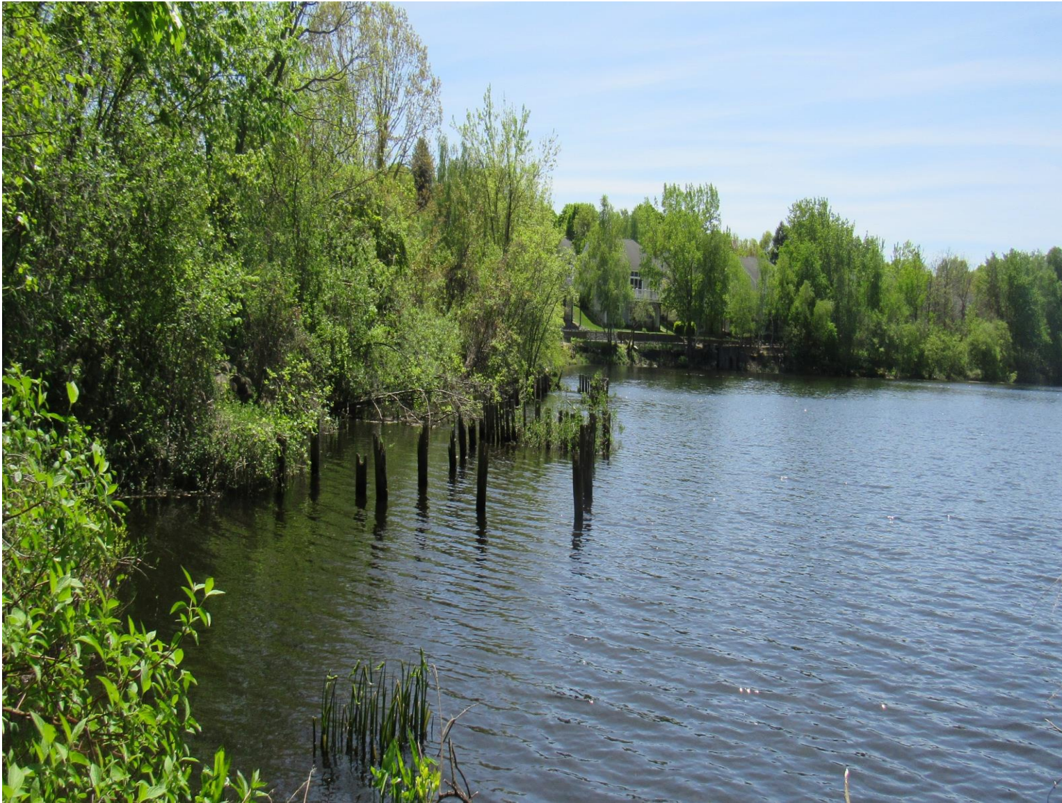
Existing View of the Spillway, looking Southeast from the bank
