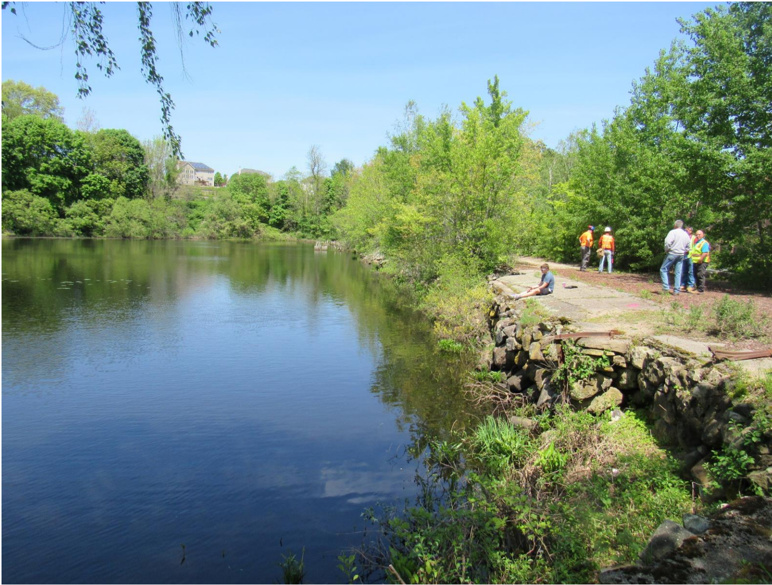
Existing View of the Top of the Dam, looking North
