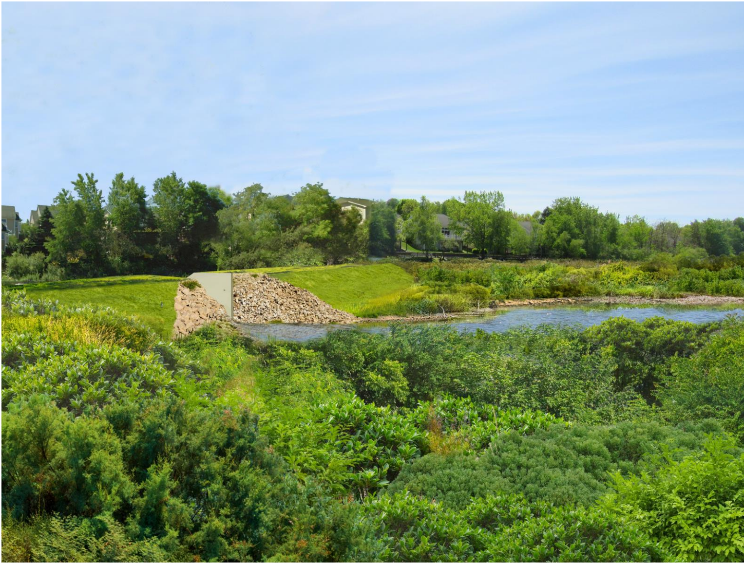
Future View of the culvert, looking Southeast from the bank
