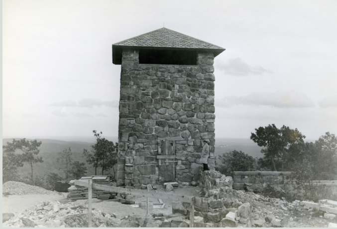
Eliot Tower construction, 1937
