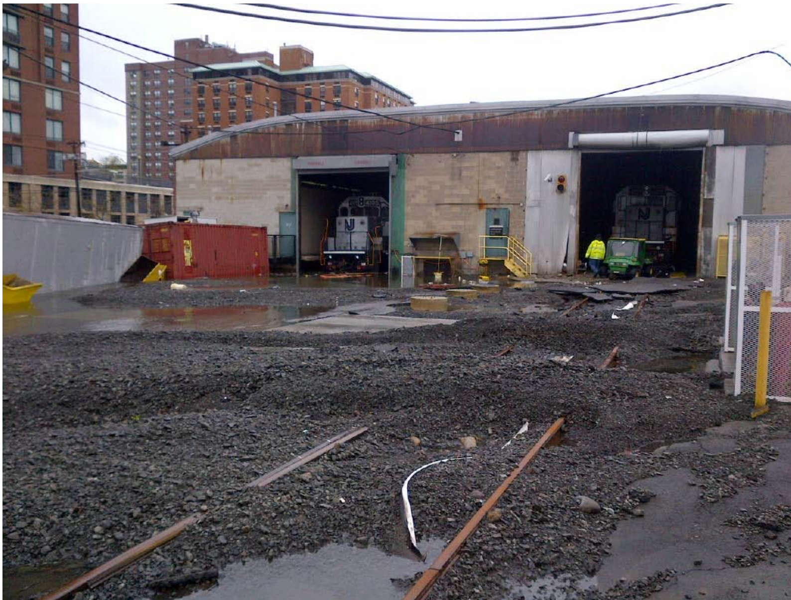
New Jersey Transit - 345 Trains damaged by flooding at the Meadowlands Maintenance Complex & Hoboken Yard totaling $120 million
