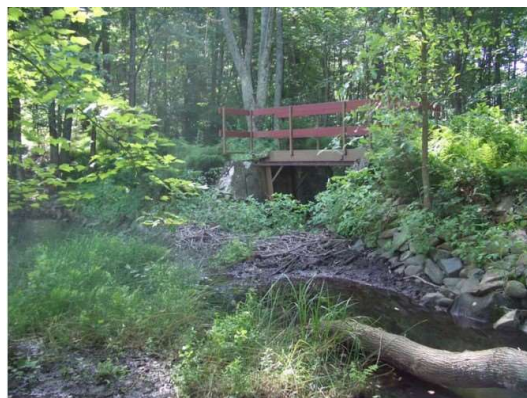
Fyfeshire Dam (prior to lowering); Source: AMEC Earth & Environmental Inc.
