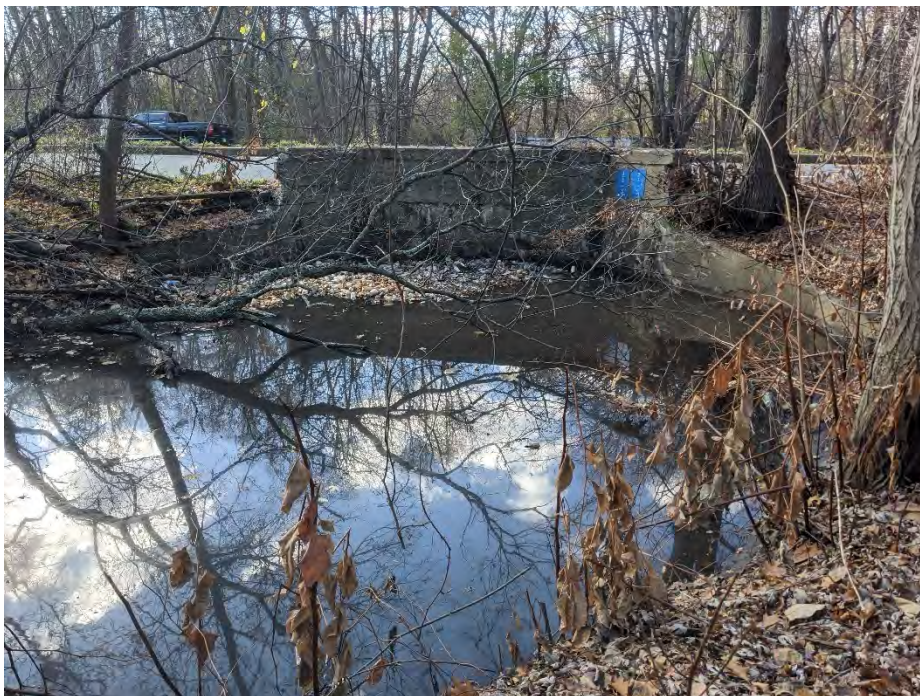
Figure 2: Existing Stream Channel and 13.5' x 6.5' Culvert (facing Morton St)
