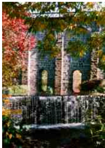
Canton Viaduct and Factory Pond on the East Branch
