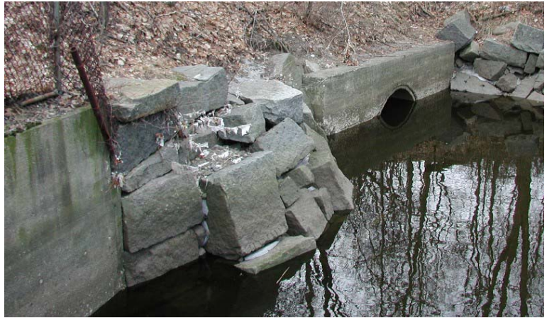
Right culvert (4 foot diameter)
