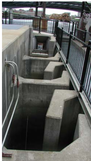
Vertical slot fishway at Charles River Locks
