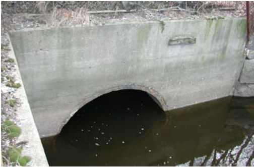
Left culvert (6 foot diameter)
