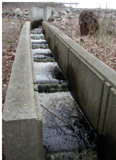
Fishway at Triphammer Pond Dam
