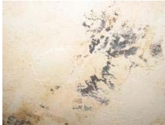
705 Family Housing Development 115 Boardman Street, Apt. #2, Building Exterior Paint Peeling on Rotted Wood
