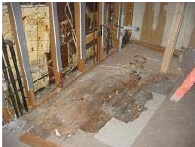
705 Family Housing Development 25 Bowdoin Street Floor is Damaged, Wall Paneling is Missing, Pipes and Wires are Exposed in Kitchen
