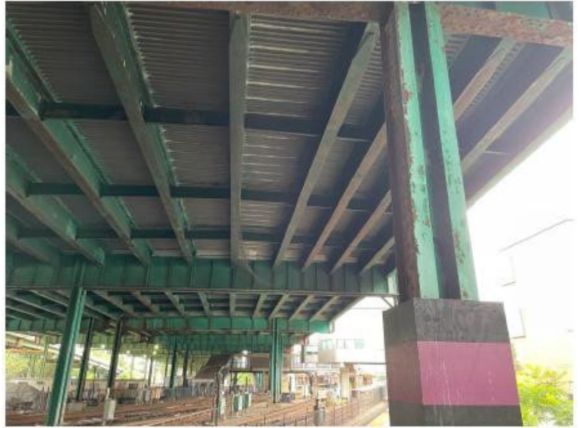
Existing conditions: bridge deck deficiencies
