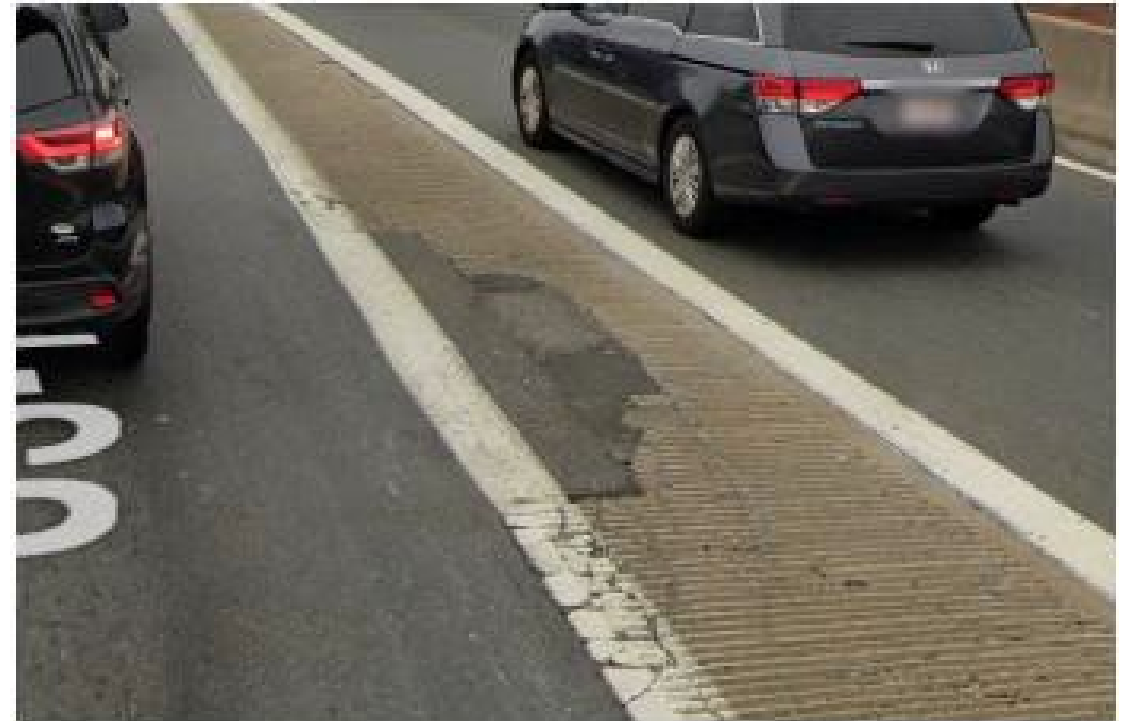
Existing conditions: typical wearing surface deficiencies
