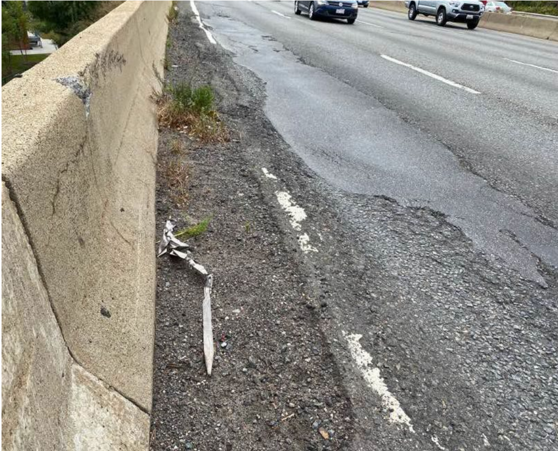
Existing conditions: Moderate cracking in southbound lane with heaving
