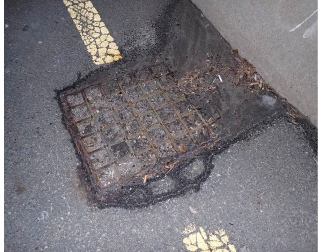
Clogged catch basin (dirt & debris)–east parapet
