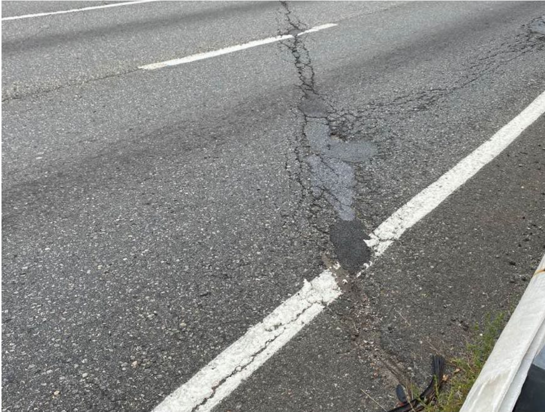
Typical transverse cracking over south abutment
