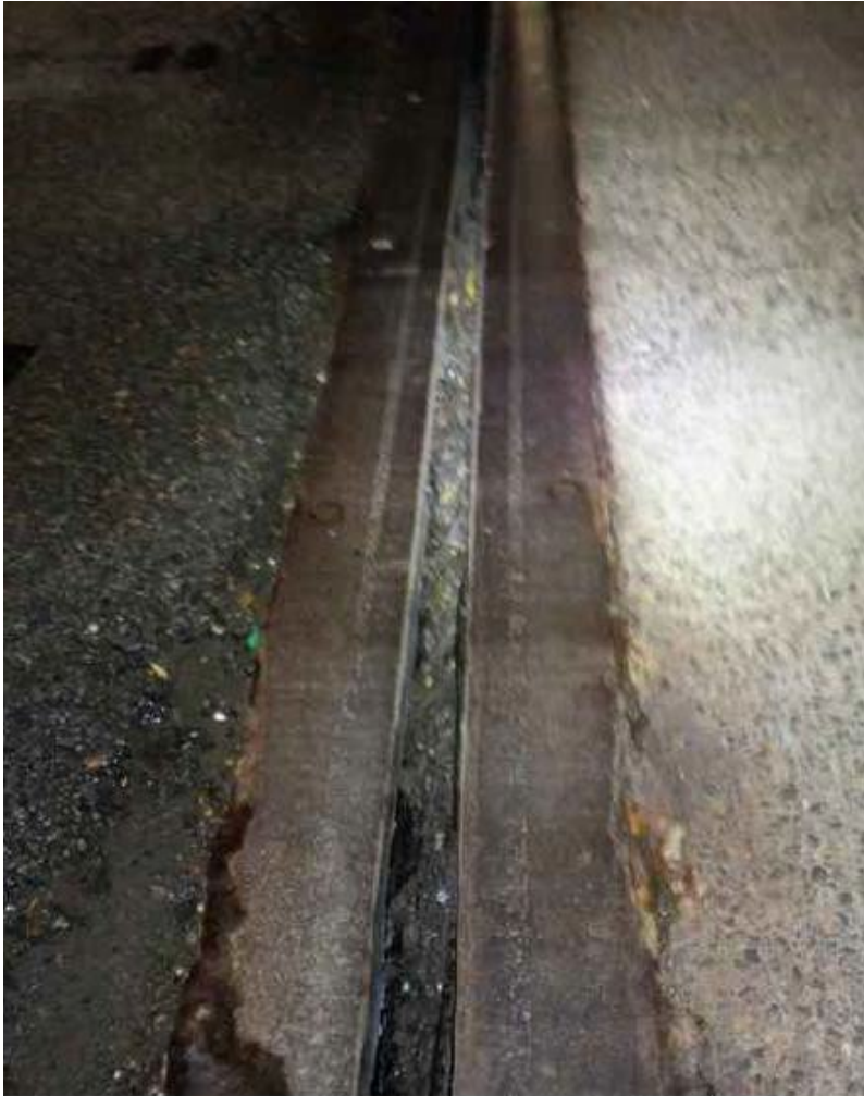
Rusted joint armor and depressed joint seal
