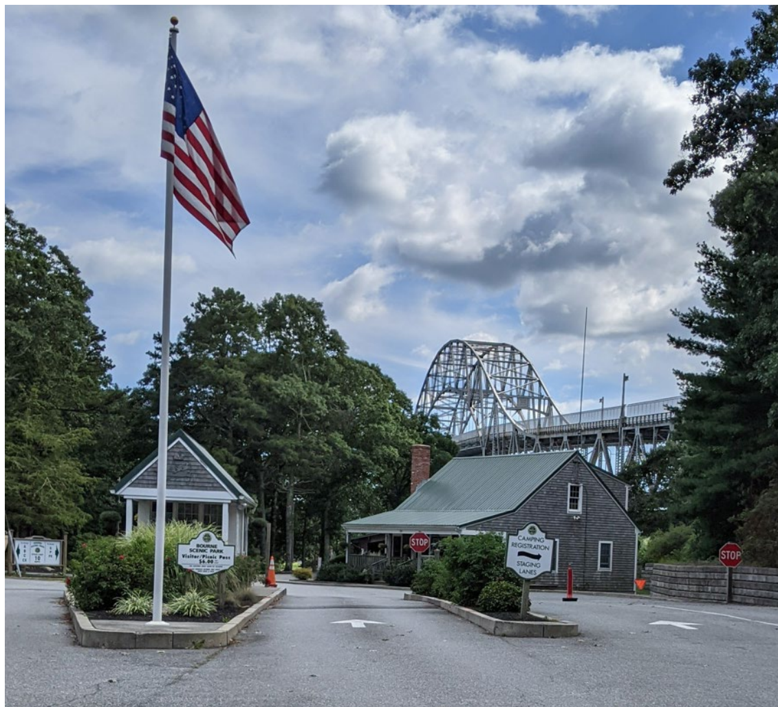
Existing BRA Office Complex
