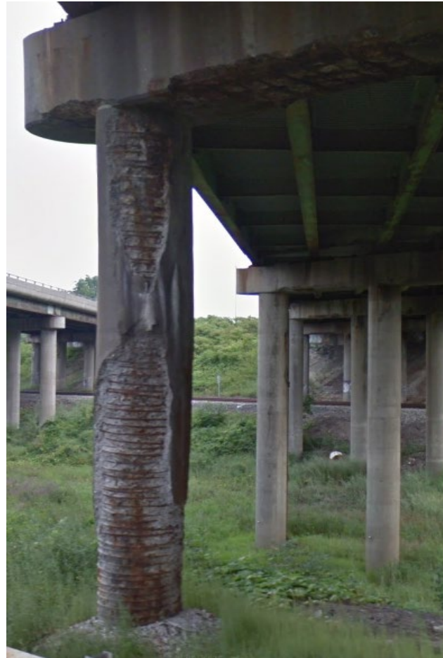
Excessive spalling
