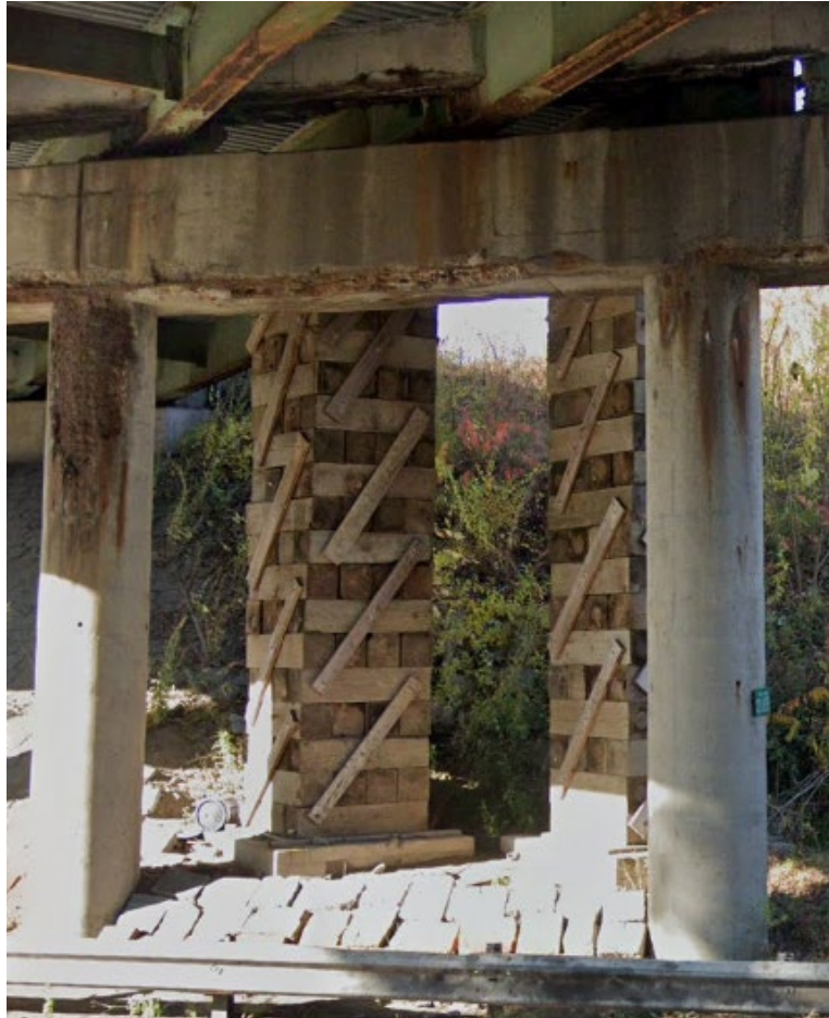
Wood cribbing installed
