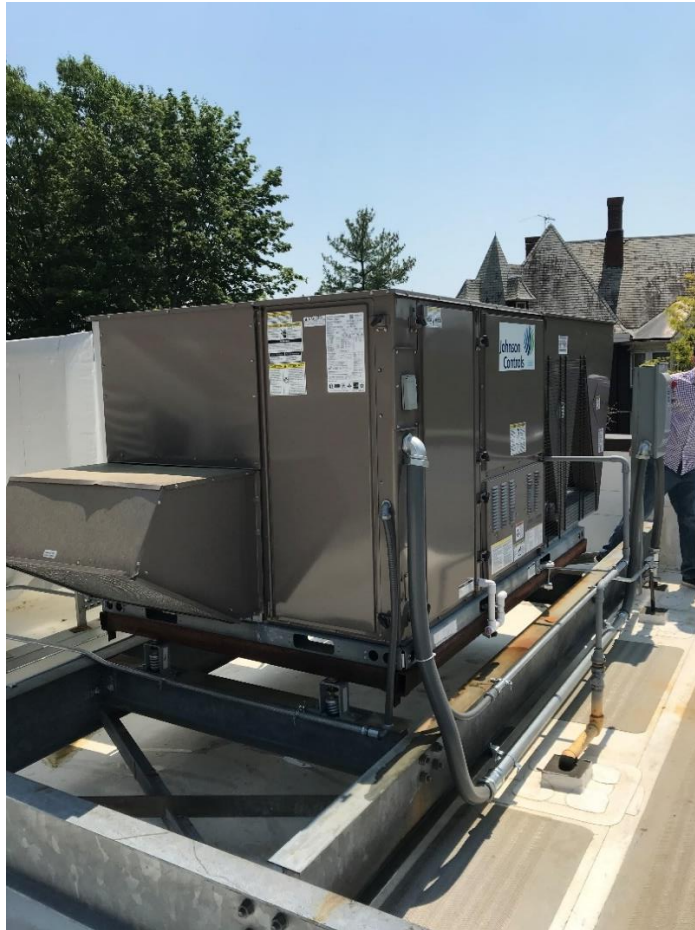
Photo 1 – Representative Roof Top Unit (RTU)
