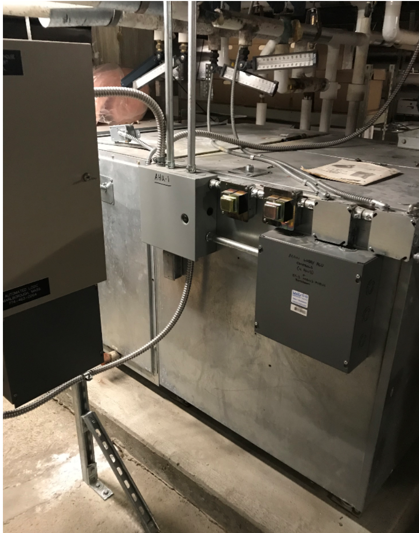
Photo 2 – Representative Air Handling Unit (AHU)
