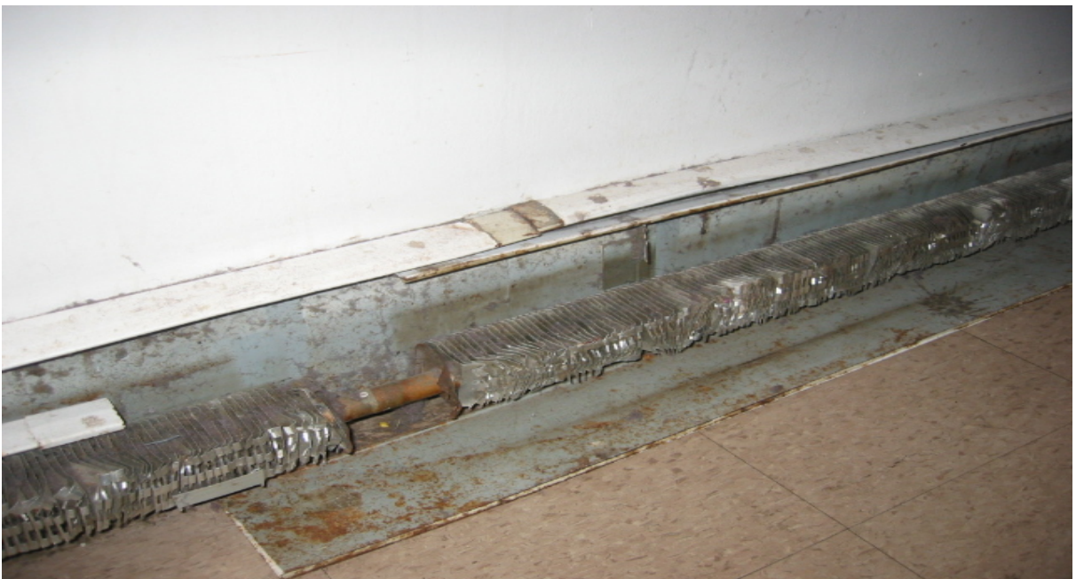
705-1 Family Housing Development Scattered Site, 19 Golden Circle Unit – Broken Electrical Heating Baseboards
