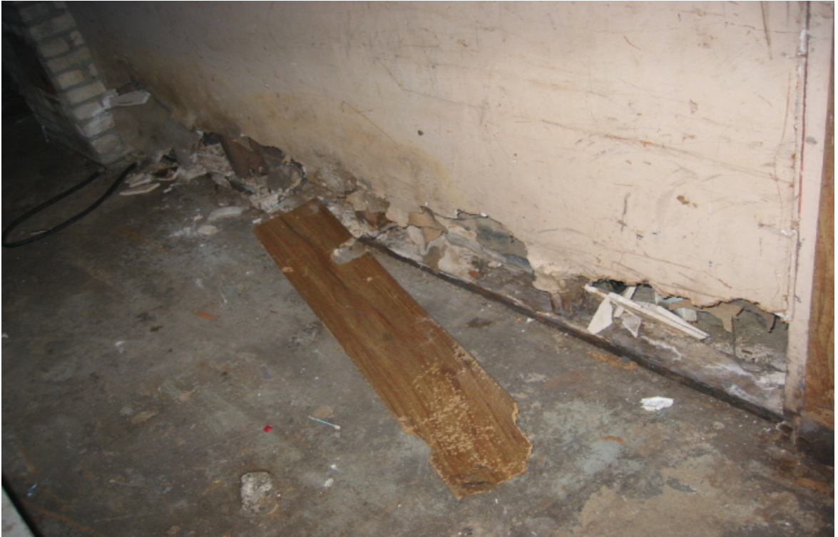
200-2 Family Housing Development, Washburn Heights, 32 Clifford Avenue Cellar – Crumbling Foundation
