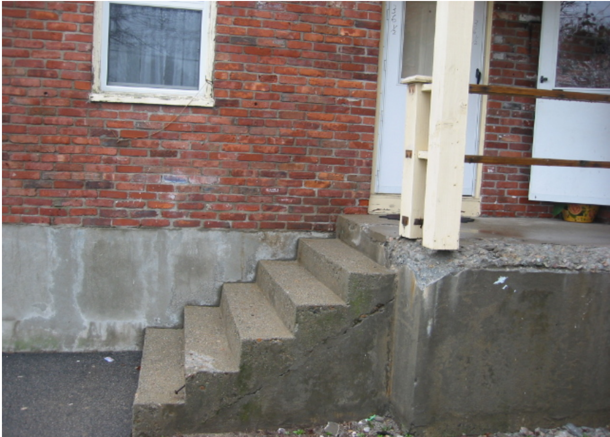
200-2 Family Development, Washburn Heights, 38 Clifford Avenue Building Exterior – Crumbling Concrete Front
