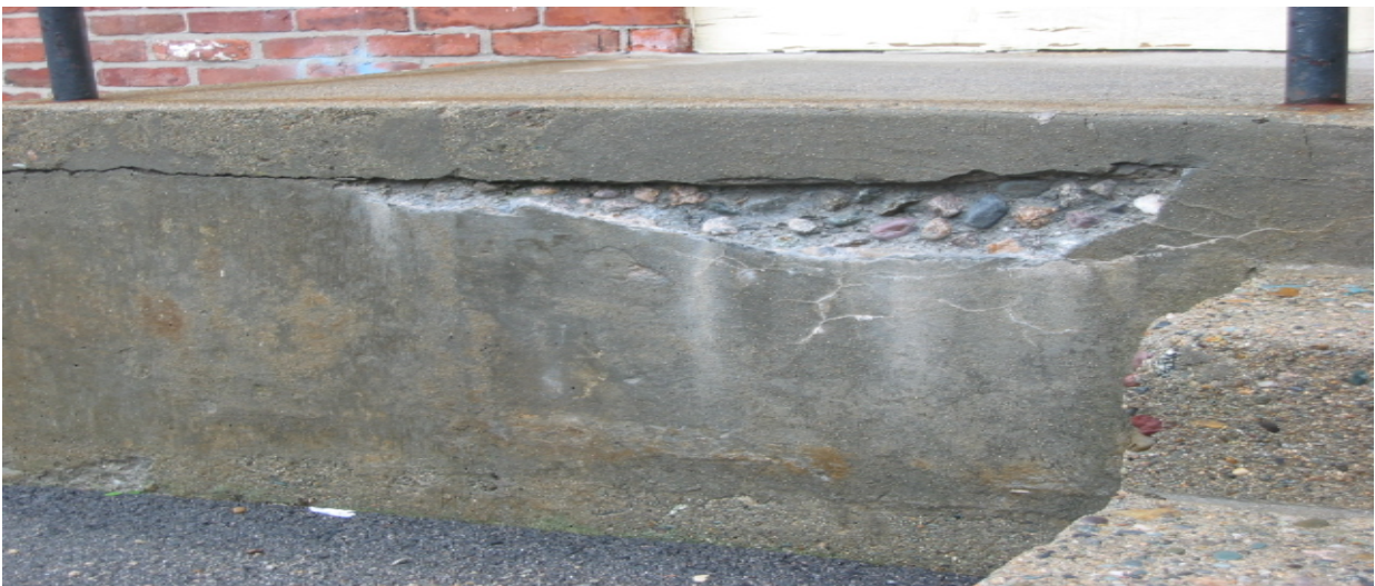
200-2 Family Development, Washburn Heights, 38 Clifford Avenue Building Exterior – Crumbling Concrete Front
