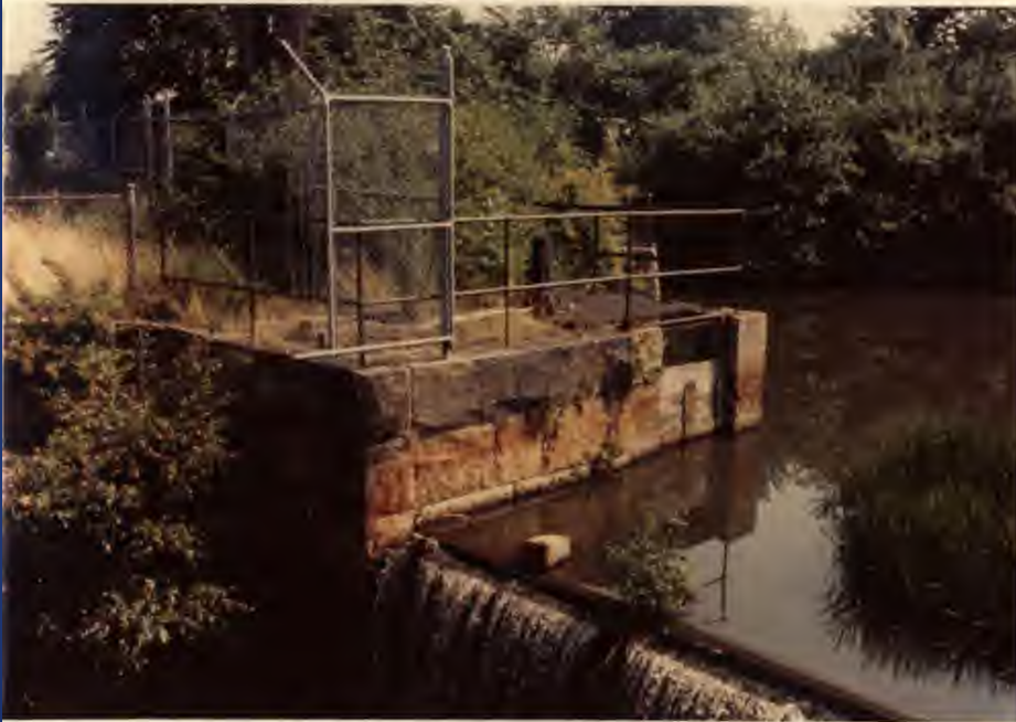
NO. 2 VIEW OF SOUTH ABUTMENT SHOWING ABANDONED INTAKE STRUCTURE
