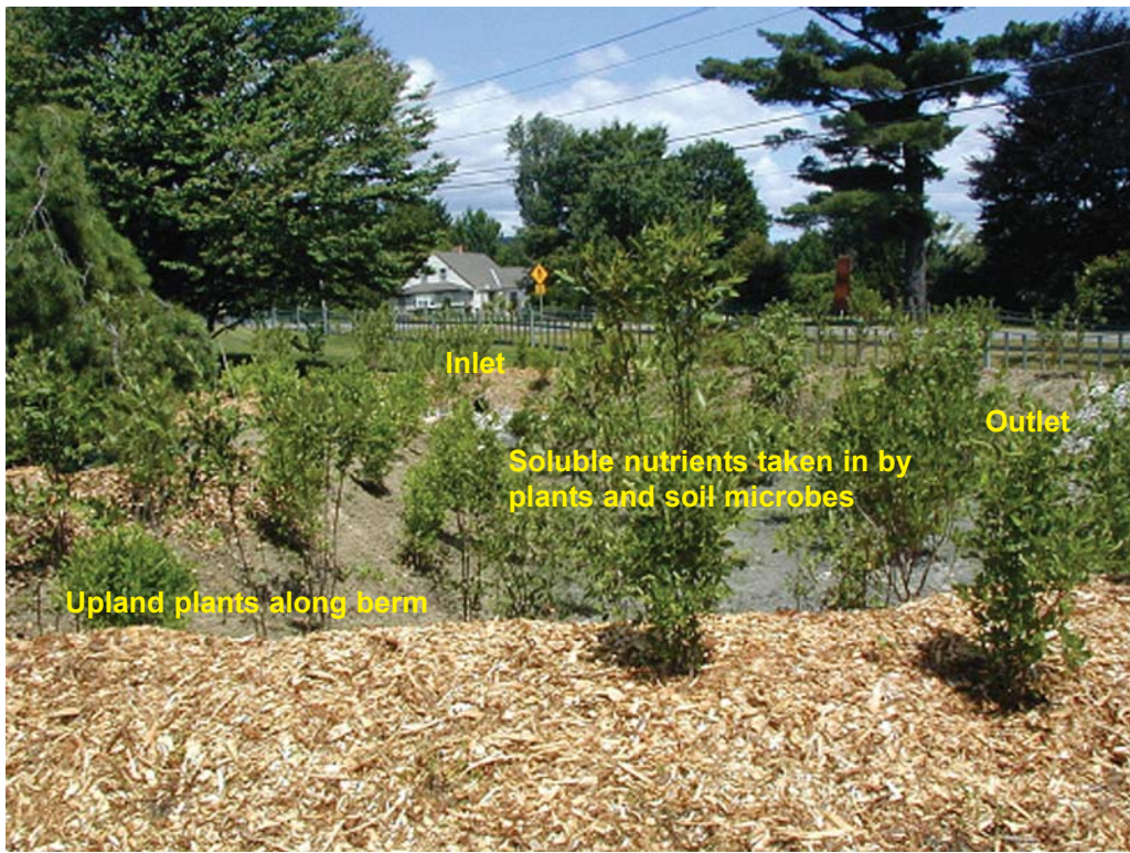
Most storm drain systems discharge untreated runoff directly into the nearest water body in older lakeside neighborhoods. Detention basins can be retrofitted into existing stormdrain systems to capture pollutants.
