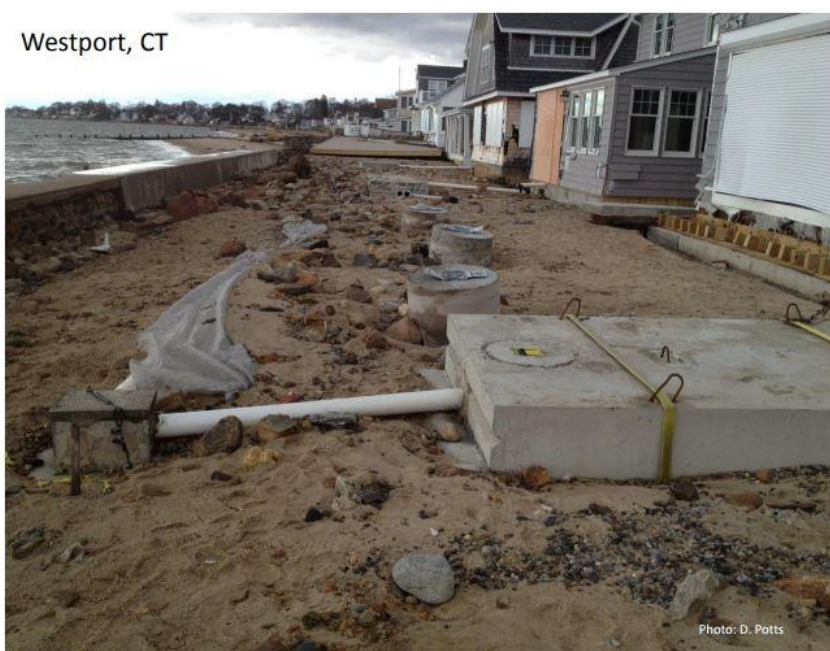
Figure 22 Exposed septic system after coastal storm, CT.
