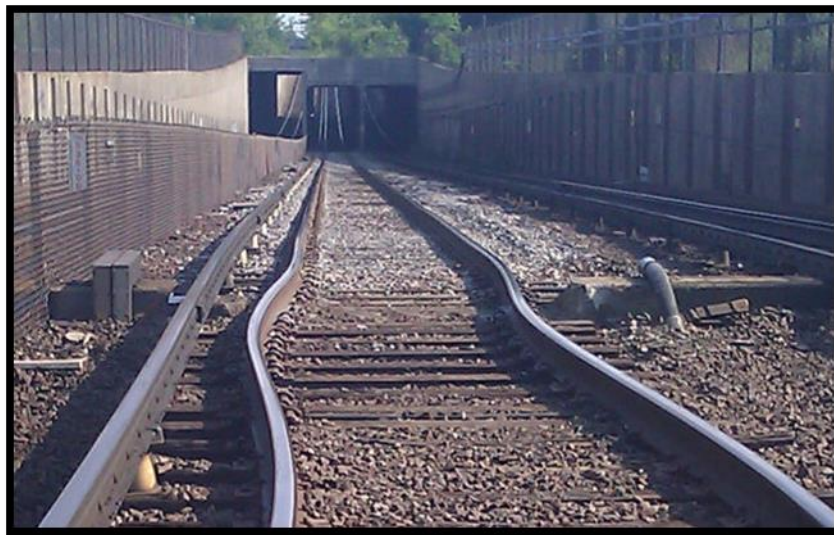
Figure 28 Heat kink on MBTA track.
