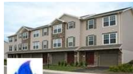
Natural Gas Heat
