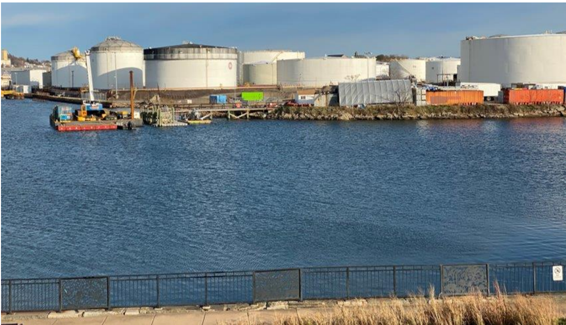
Figure 8 – View of oil terminal in Chelsea Creek DPA
