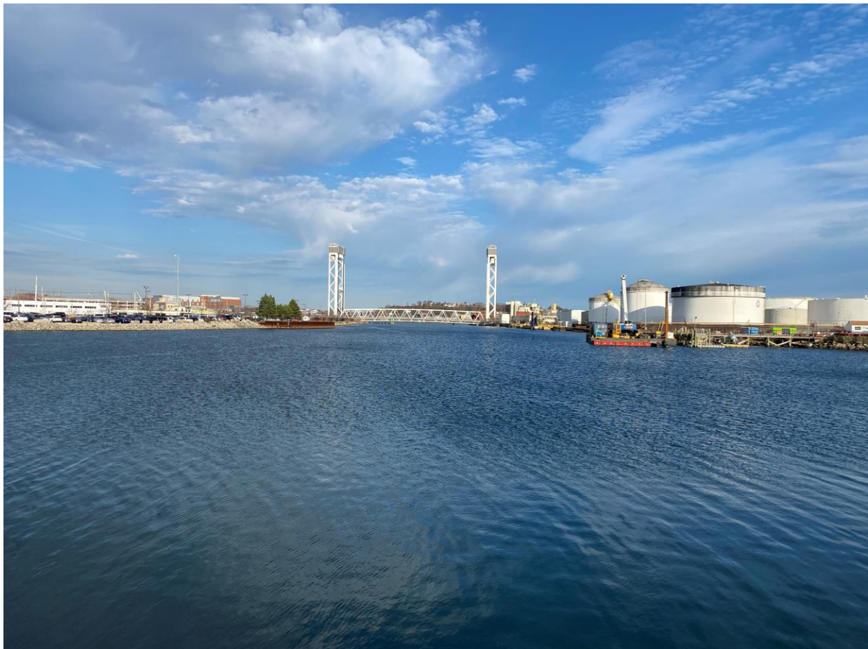
Figure 2 – View of the Chelsea Creek DPA facing northeast
