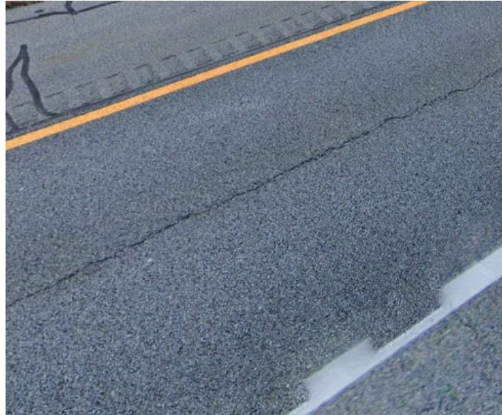
Existing pavement conditions necessitate preservation action (longitudinal pavement cracking shown)
