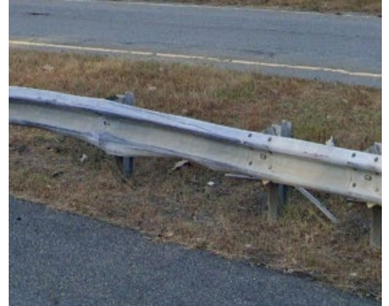
Existing guardrail systems need repair/replacement
