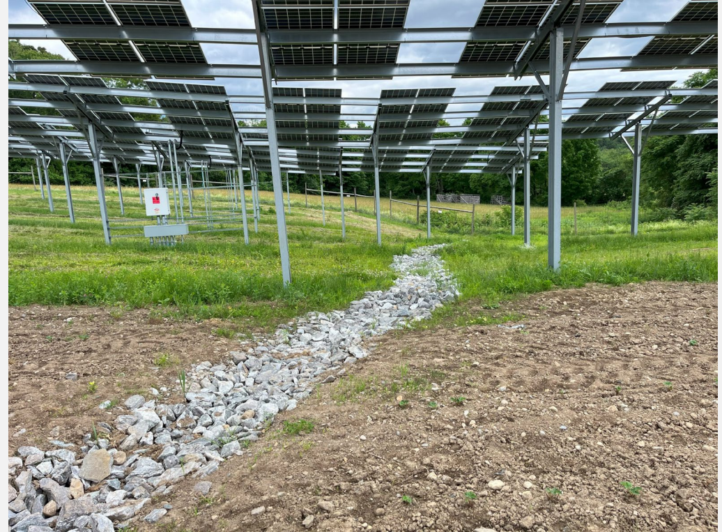
Underground Pipe and Rock Installation
