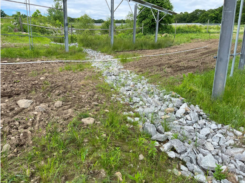
Underground Pipe and Rock Installation
