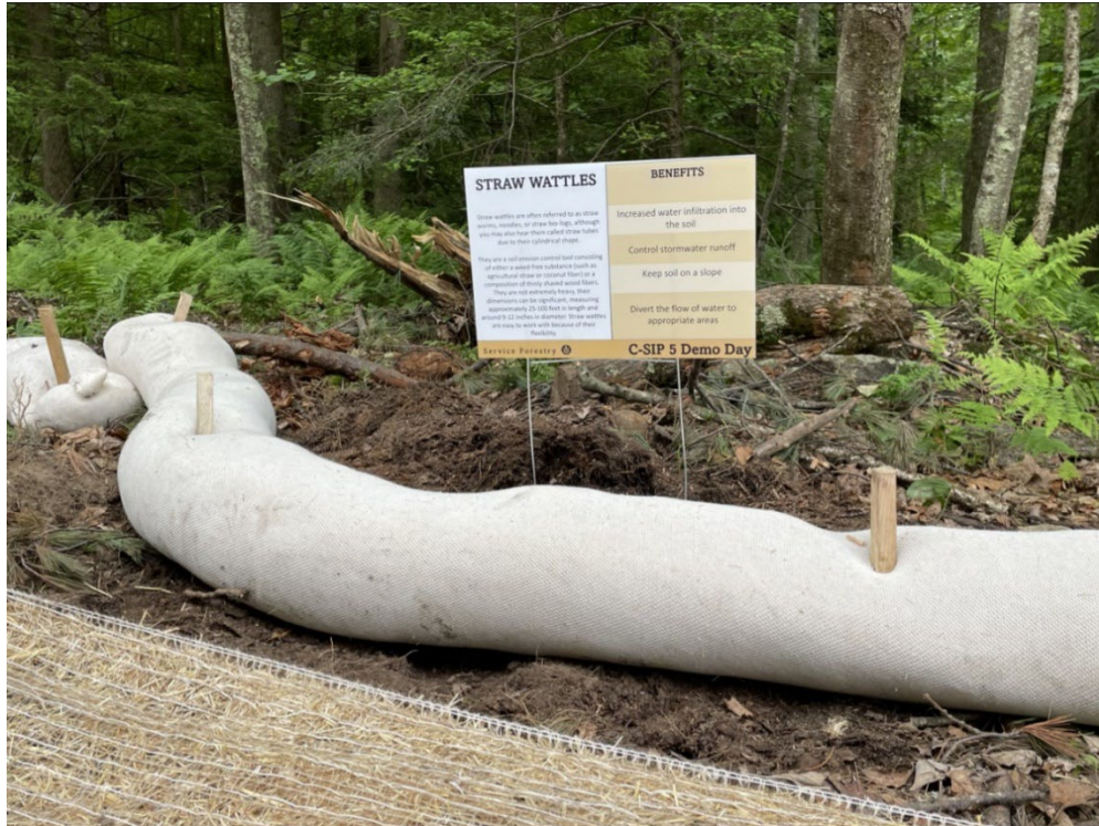
Finished Installation of a straw wattle on an active harvest. C-SIP 5 Demo day, Town of Athol. Photo credit: Sara Wisner
