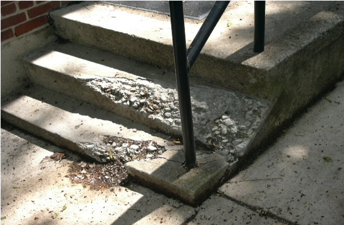
200-3 Development, 43 Lincoln Way Damaged Concrete Stairs
