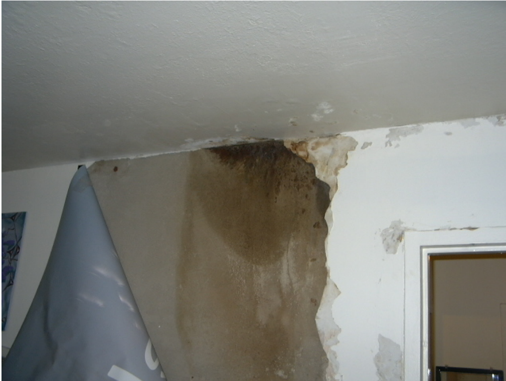
200-5 Development, 5 Jackson Gardens, #27 Mold and Water Damage on Walls and Ceiling in Bathroom
