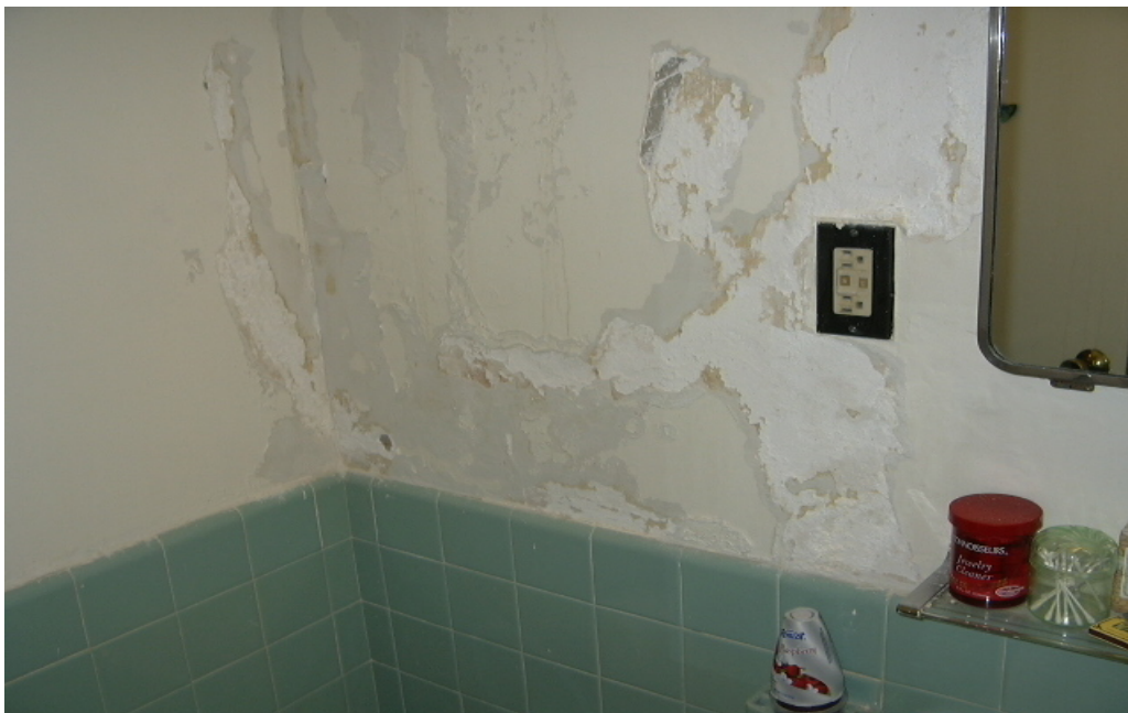
200-5 Development, 5 Jackson Gardens, #27 Mold and Water Damage on Walls and Ceiling in Bedroom
