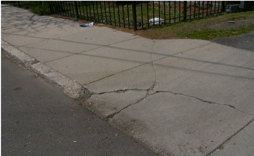
705-1 Development, 58 Willow Street Cracked and Heaved Sidewalks
