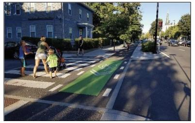
lanes, a sidewalk-level cycle track on one side of the street, and side street crossing tables (SSCTs) that carry the sidewalk and cycle track over side streets.
