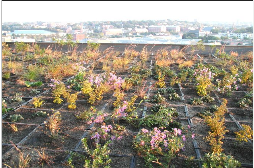
Massachusetts College of Art’s Green Roof Pilot was initiated through a $10,000 grant from the Executive Office of Energy and Environmental Affairs. Located on the 11th floor of the school’s Tower Building, the garden portion is 750 square feet of native plant species.
