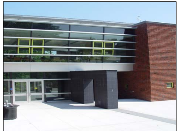
Cape Cod Community College's new Lyndon P. Lorusso Applied Technology Center was the first building constructed with Massachusetts' state funding to receive LEED ® (Gold) certification.
