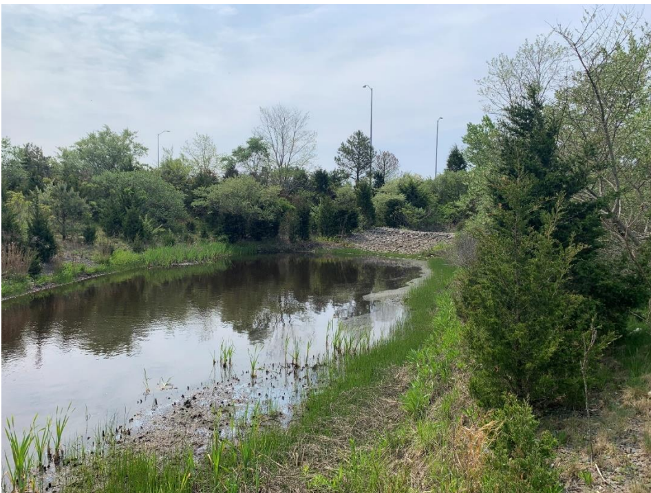
Exhibit 5-3. Stormwater Basin at State Route 3 North Off-Ramp to U.S. Route 6 West (Sagamore North Quadrant)
