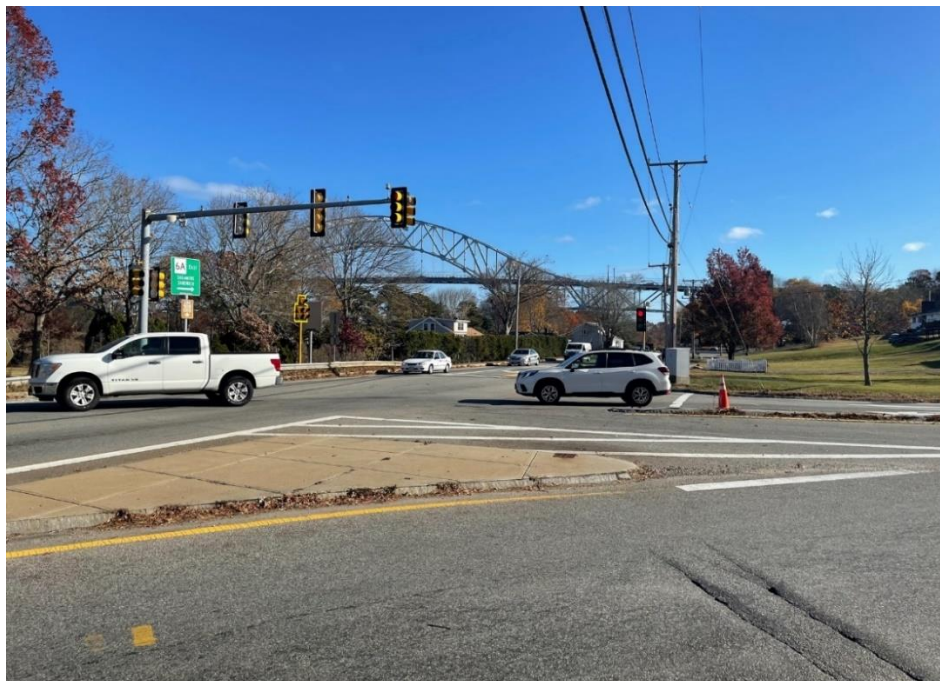
Exhibit 6-7a. Existing View from Sandwich Road at Mid-Cape Connector, facing east
