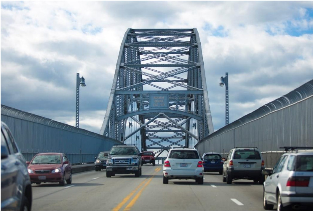
Exhibit 6-1a. Existing View from Motorist (Sagamore and Bourne Bridges)
