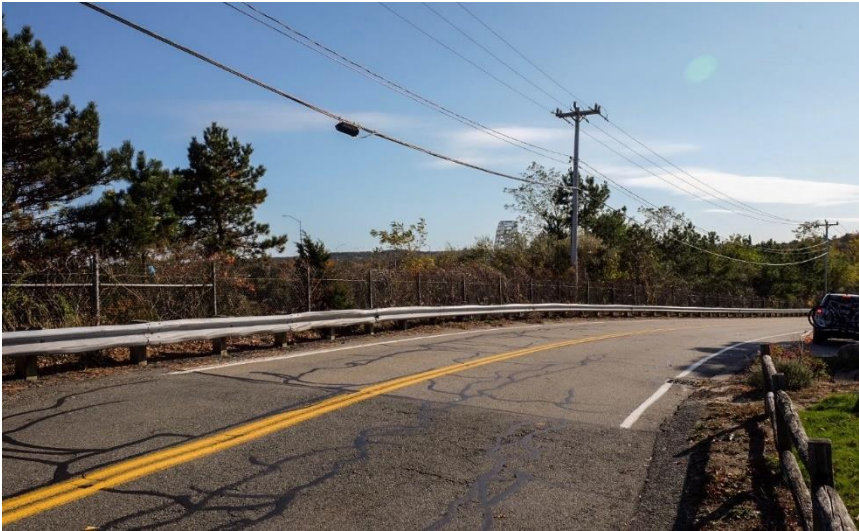
Exhibit 5-10. View of Sagamore Bridge from Church Lane at Cape Pine Road, facing south
