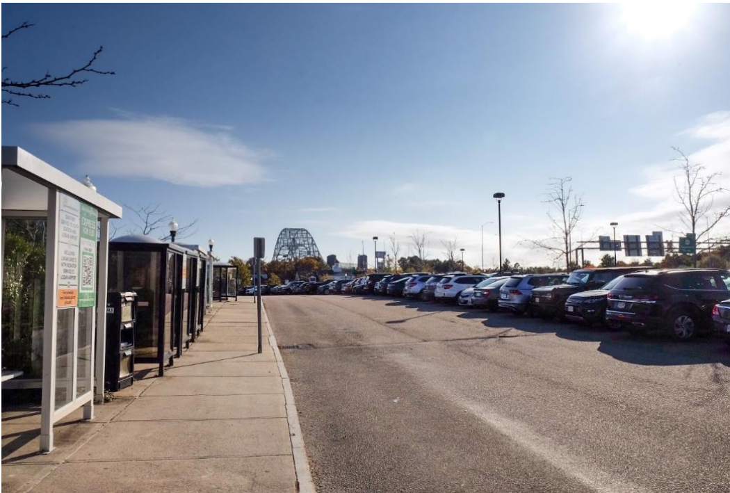
Exhibit 5-22. View of Sagamore Bridge from Bourne Park and Ride Lot, facing southwest
