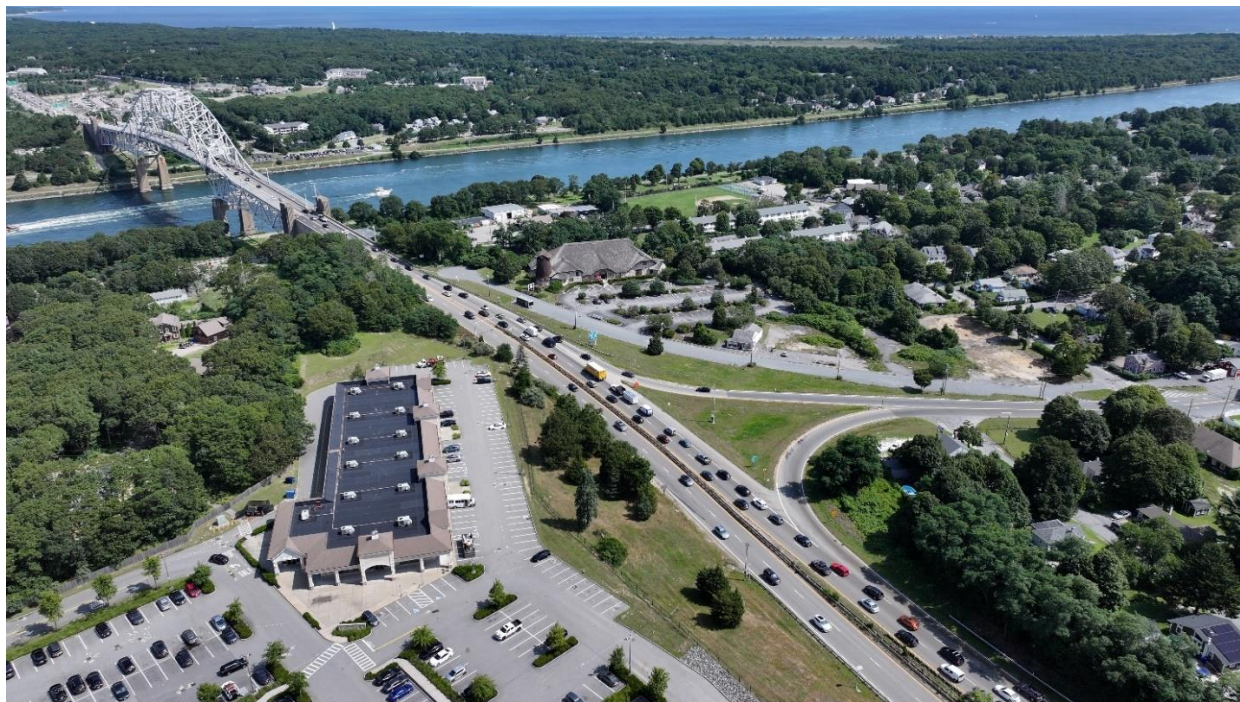
Exhibit 5-7. U.S. Route 6 facing northwest to Sagamore Bridge (Sagamore South Quadrant)
