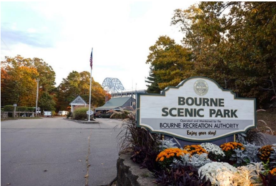
Exhibit 5-16. View of Bourne Bridge from Bourne Scenic Park entrance, facing south
