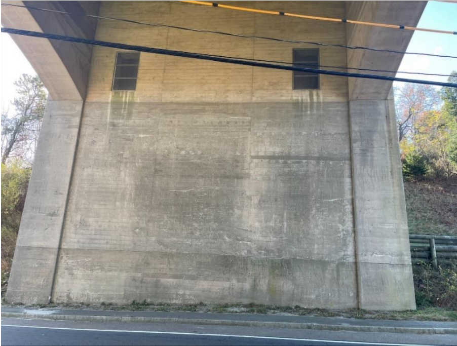
Exhibit 6-9a. Existing View from Sandwich Road at Sagamore Bridge South Abutment, facing south
