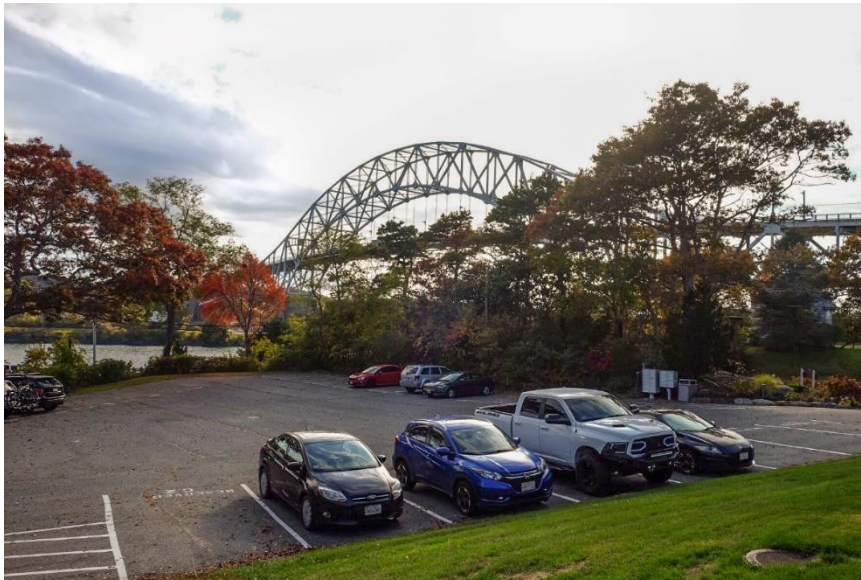
Exhibit 5-12. View of Sagamore Bridge from Hunters Brook Condominiums, facing southwest
