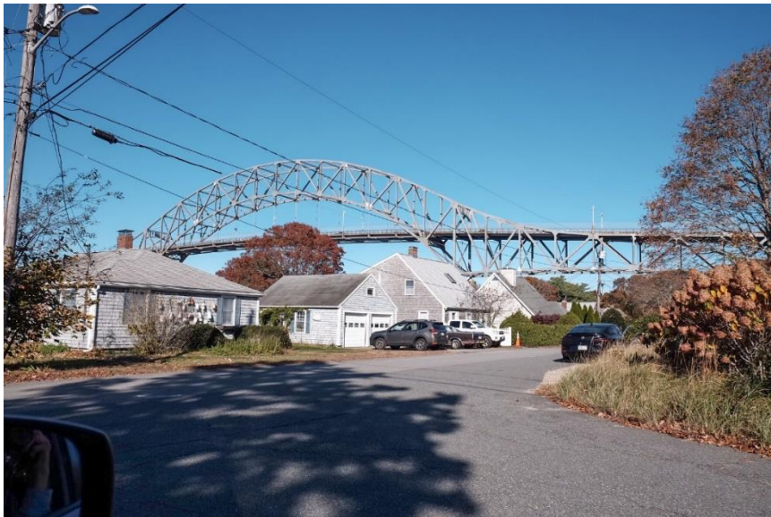
Exhibit 5-13. View of Bourne Bridge from Winslow Street, facing northeast
