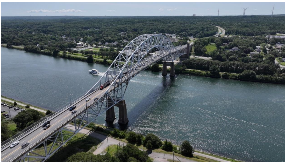
Exhibit 5-1. View of Sagamore Bridge, facing southeast
